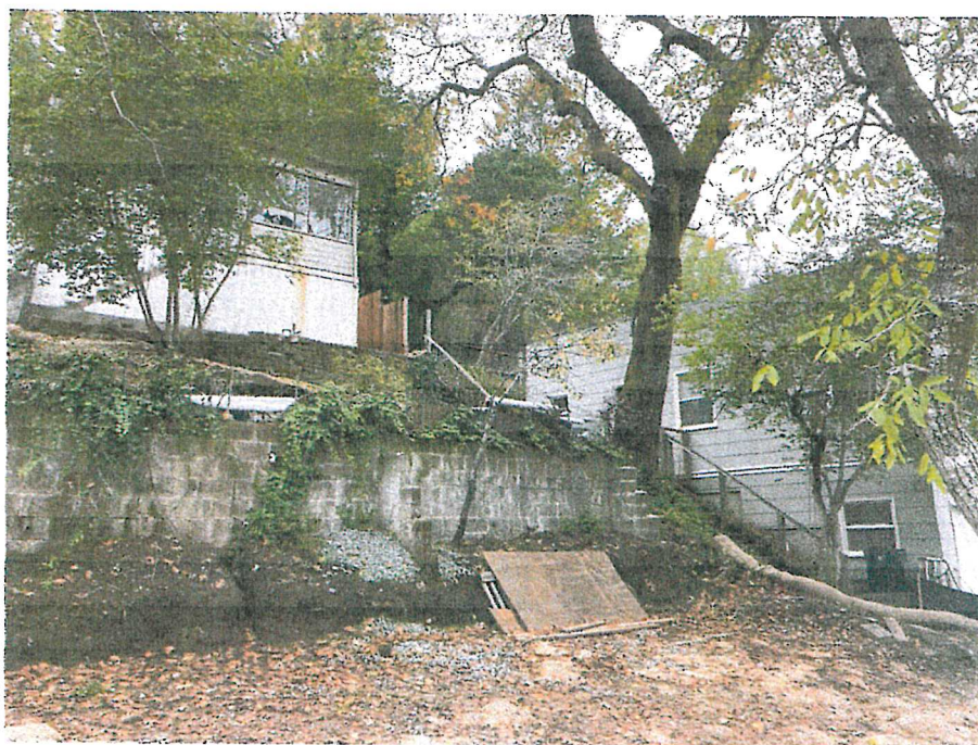
PHOTOGRAPH NO. 2: Subject Heritage oak tree T1 (center) and its proximity to existing retaining wall.
