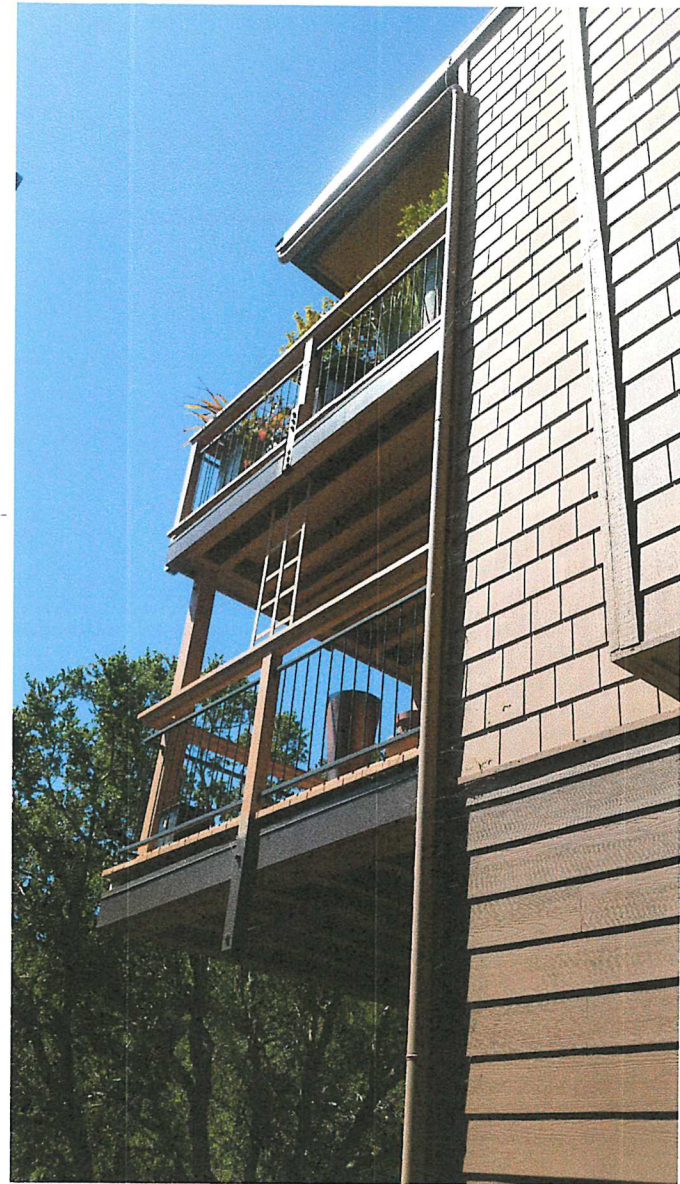
VIEW OF EAST WALL 81 PINE DRIVE-DECKS
