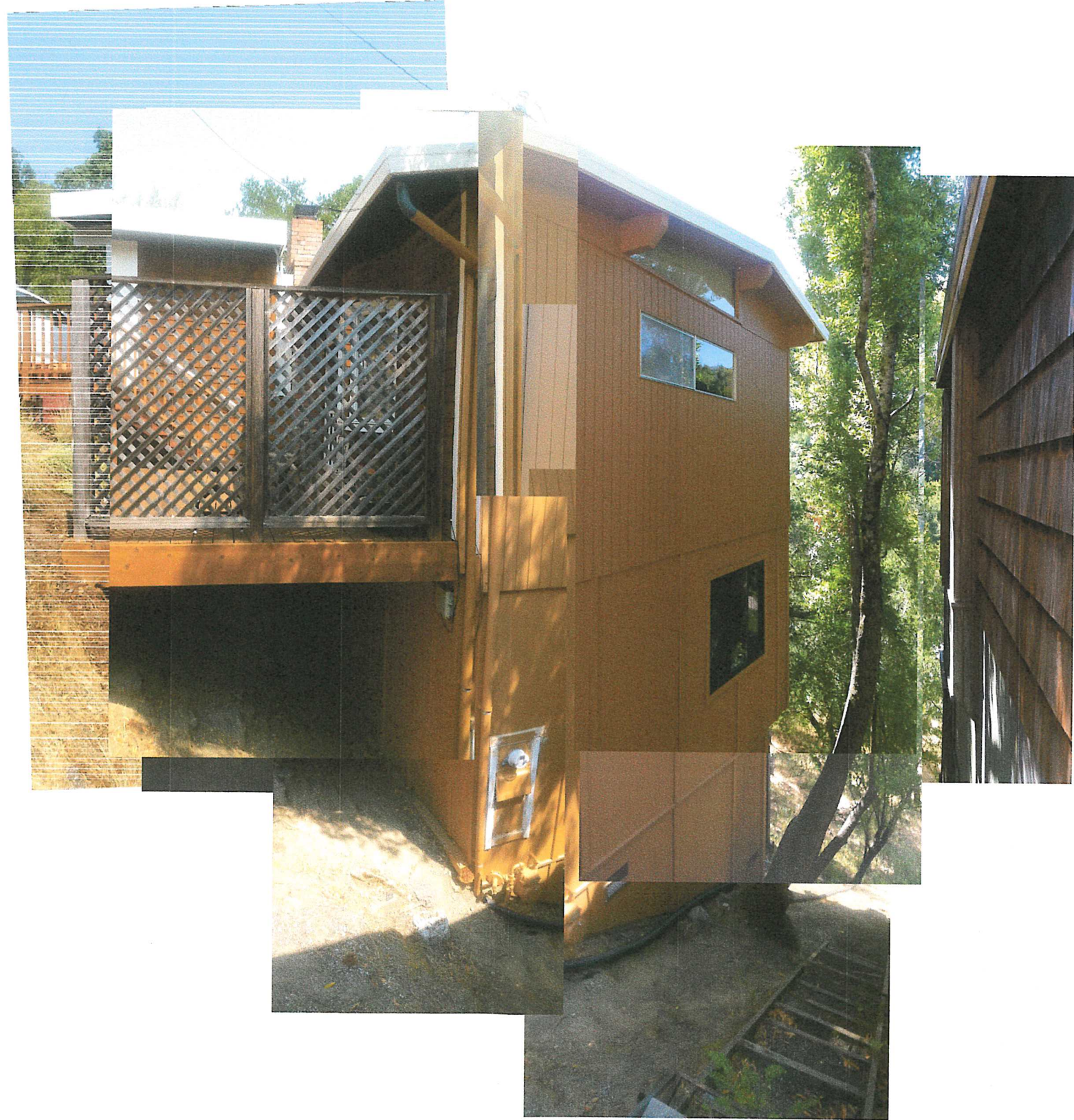
VIEW OF WEST WALL 69 PINE DRIVE
