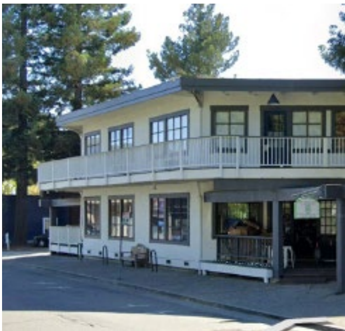
Figure x.03.050.5: Example of upper level circulation encroaching over the sidewalk
