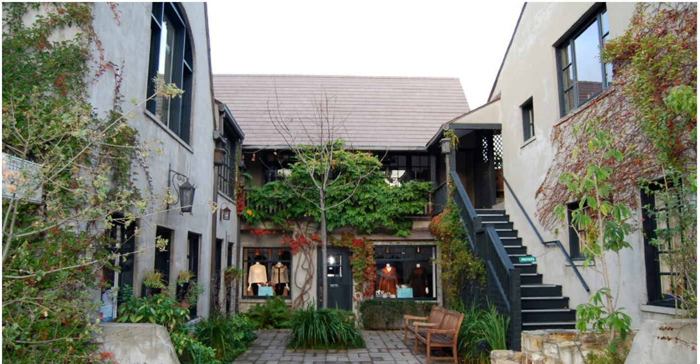
Example of a Forecourt with Shopfronts
