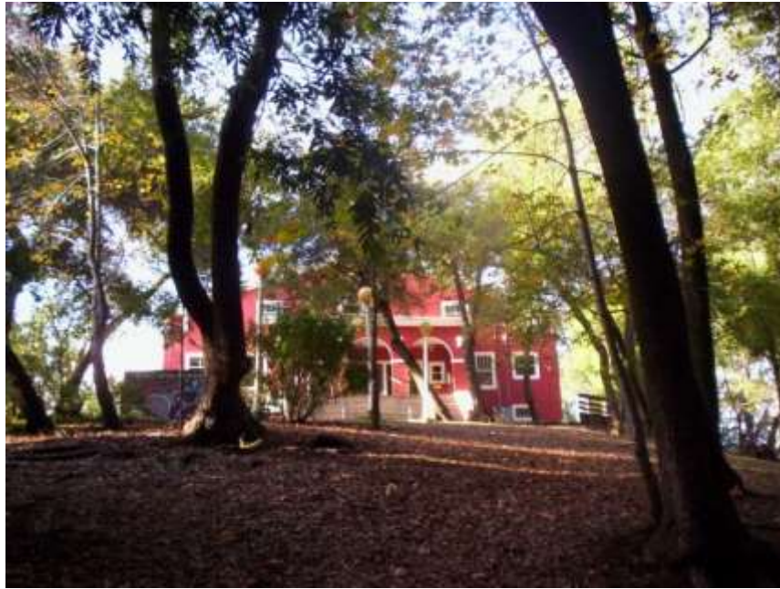
Exterior of building
