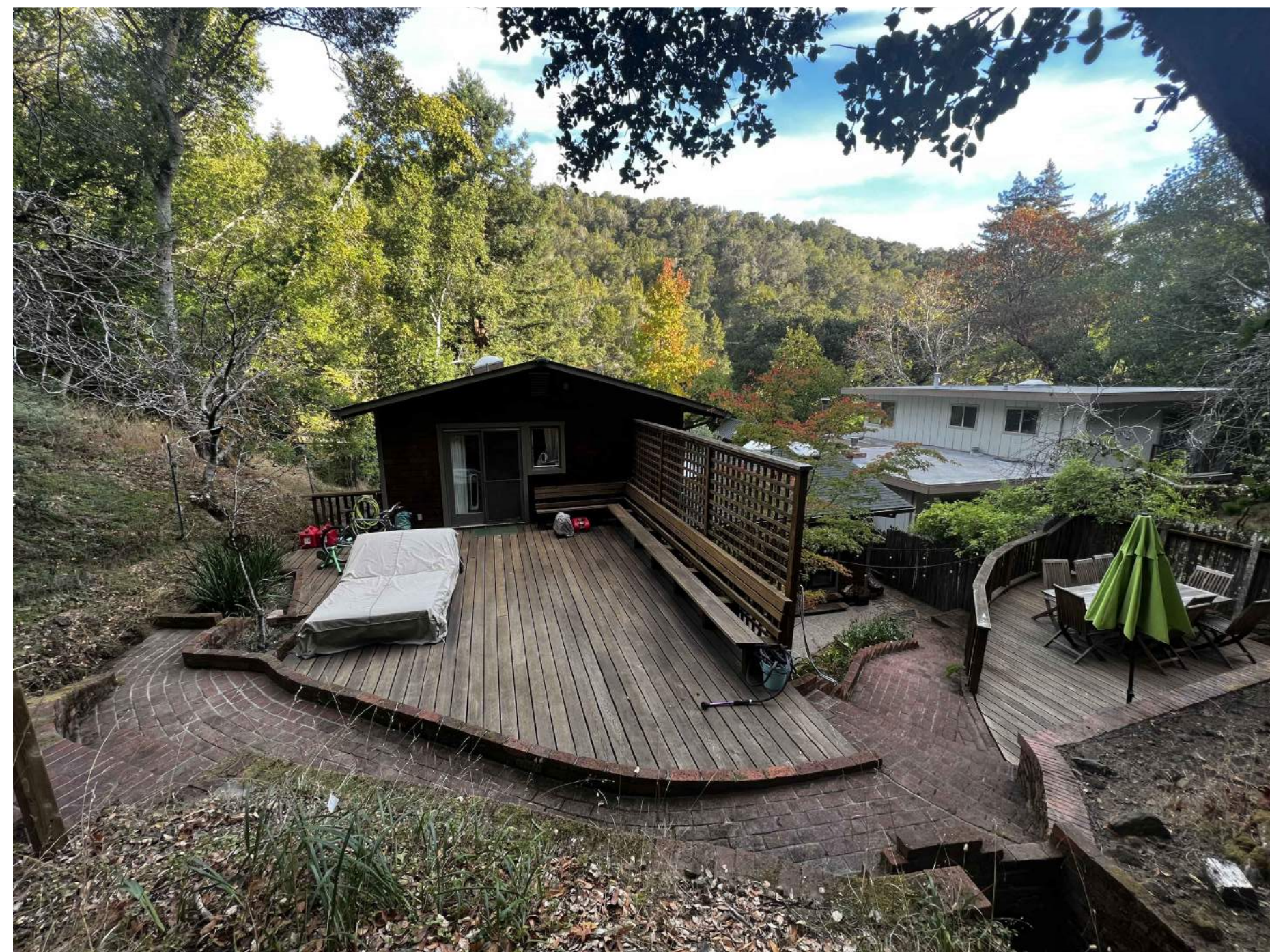
EXISTING DECK PHOTO 2 SCALE 1/4" = 1'-0" A3.2
