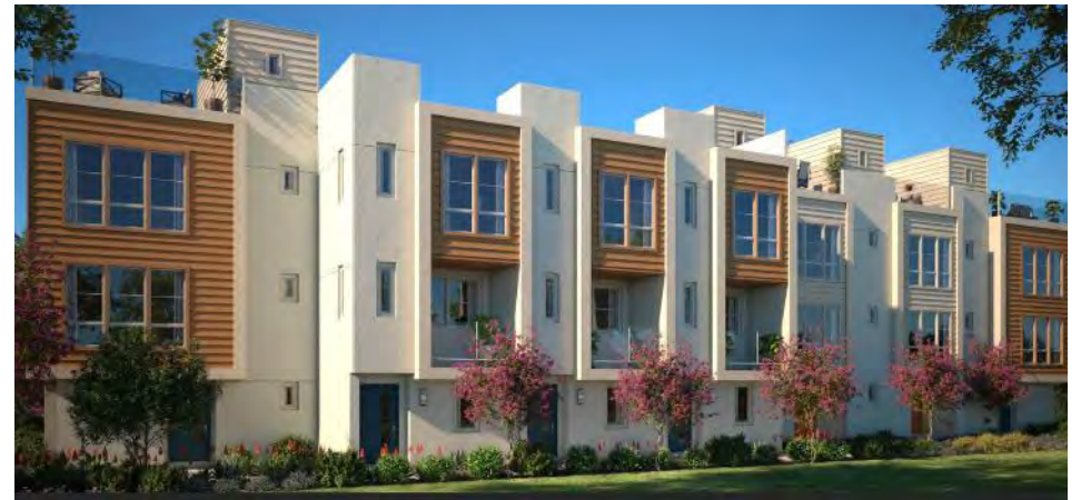
Built Project Exterior
