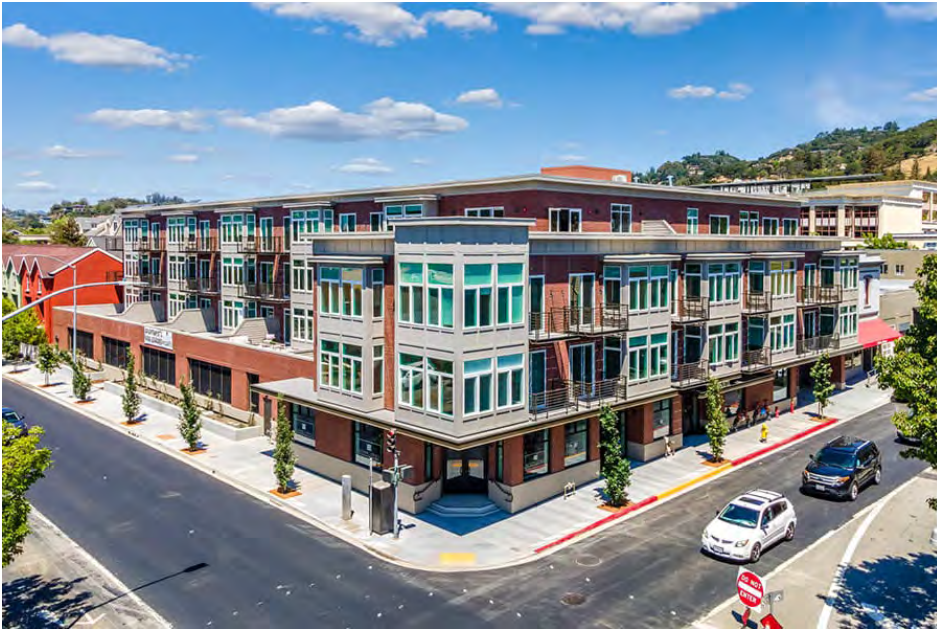
Existing Building Facade
