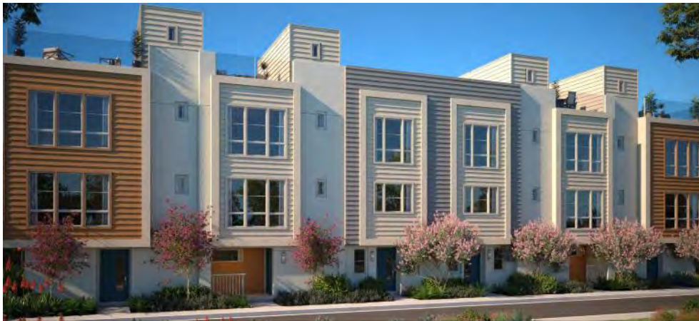
Built Project Exterior
