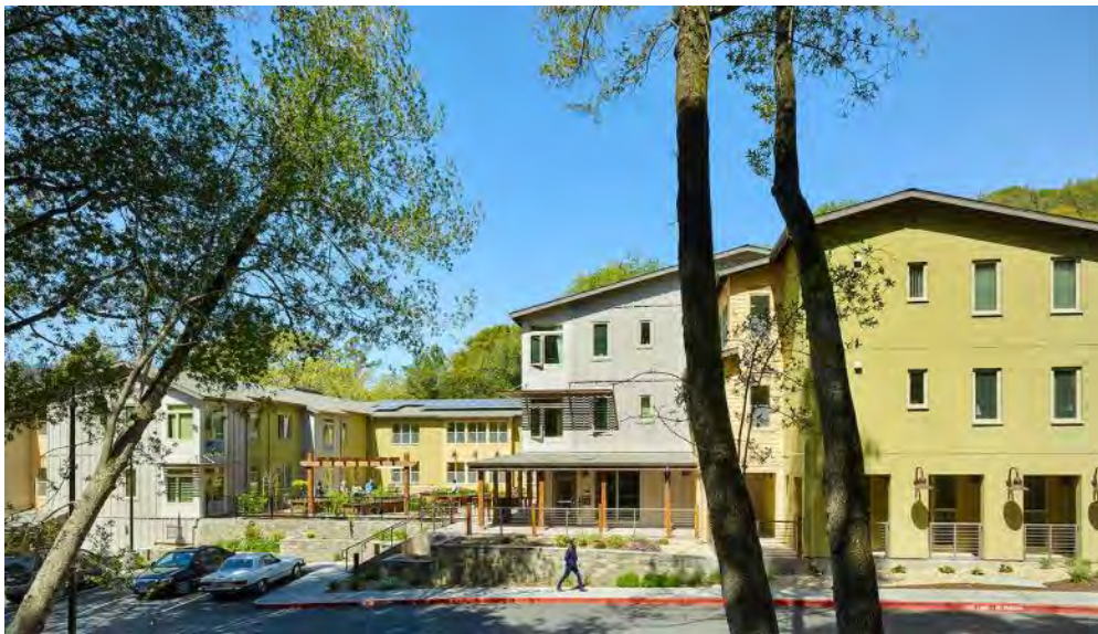
View of Existing Building from Street
