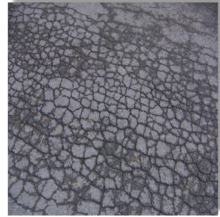
Alligator Cracking
