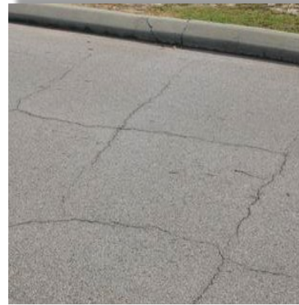
Block Cracking
