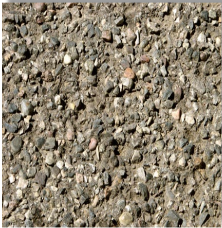
Weathering or Raveling
