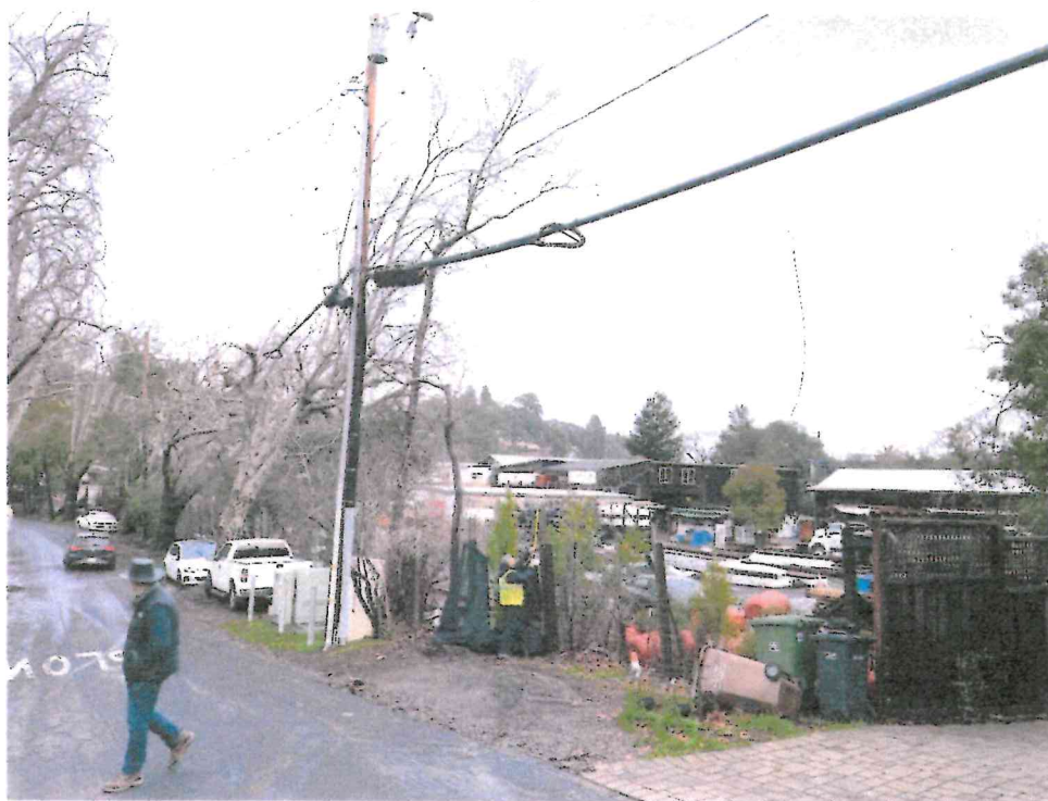
1 EXISTING CONDITIONS -VIEW FROM SPRUCE, TOP OF HILL Scale: AS INDICATED
