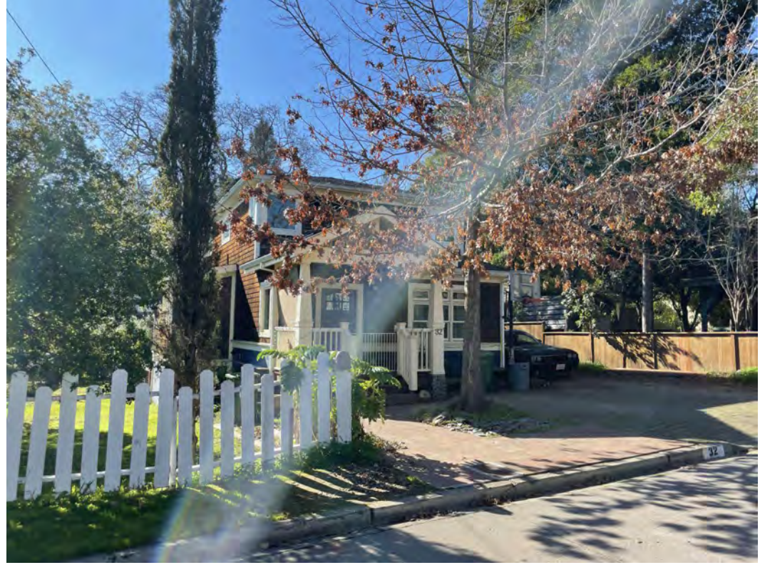
32 HILL AVE - NORTHEAST VIEW
