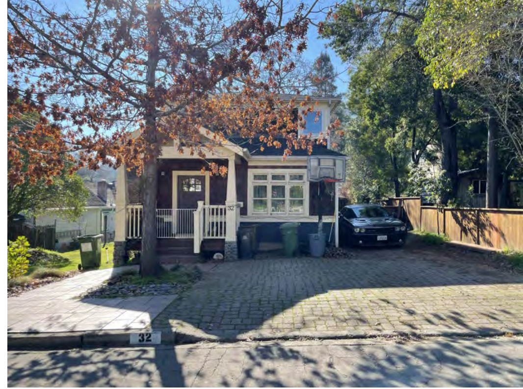
32 HILL AVE - NORTH VIEW
