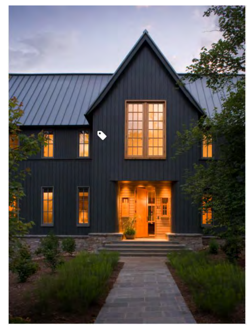
STANDING SEAM METAL ROOFING & BLUESTONE PAVERS
