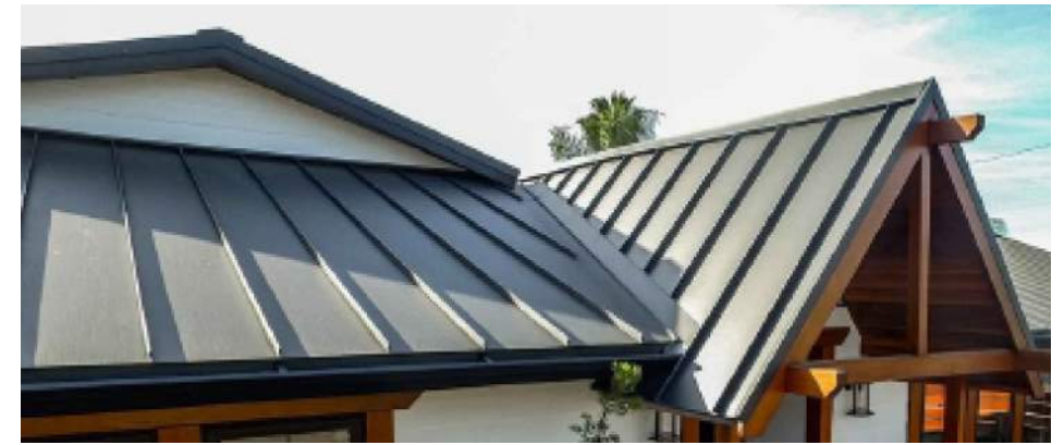
STANDING SEAM ROOF
