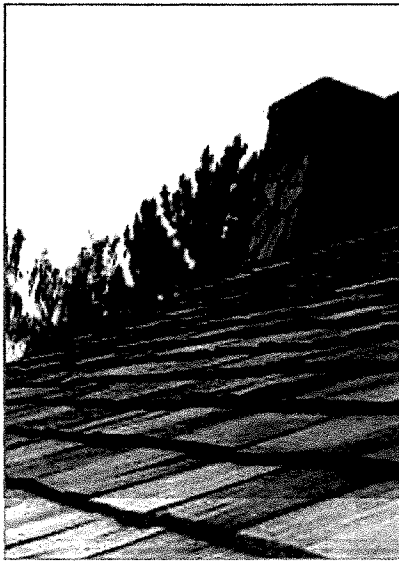
Wood shingle roof Courtesy of Gutter Glove
