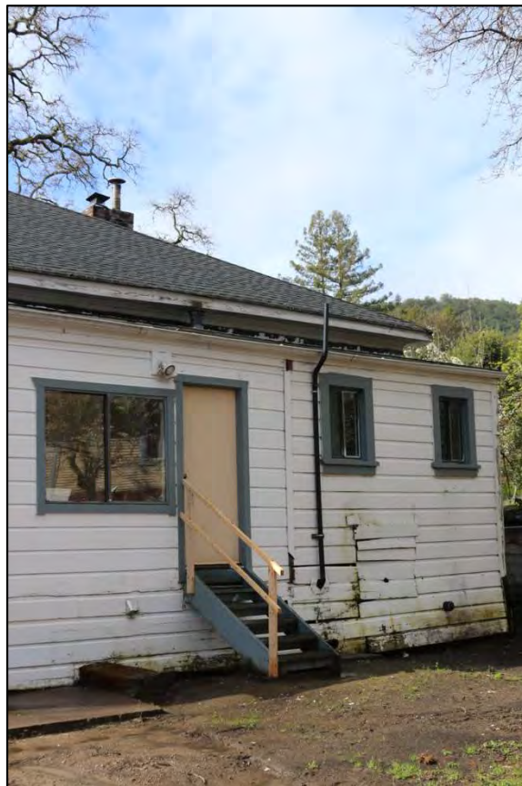
Figure 22: North elevation, NW corner
