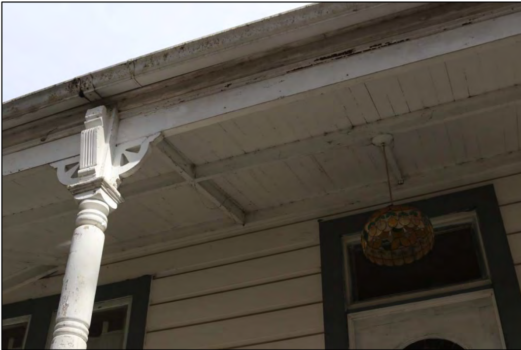
Figure 8: South elevation, roof of porch
