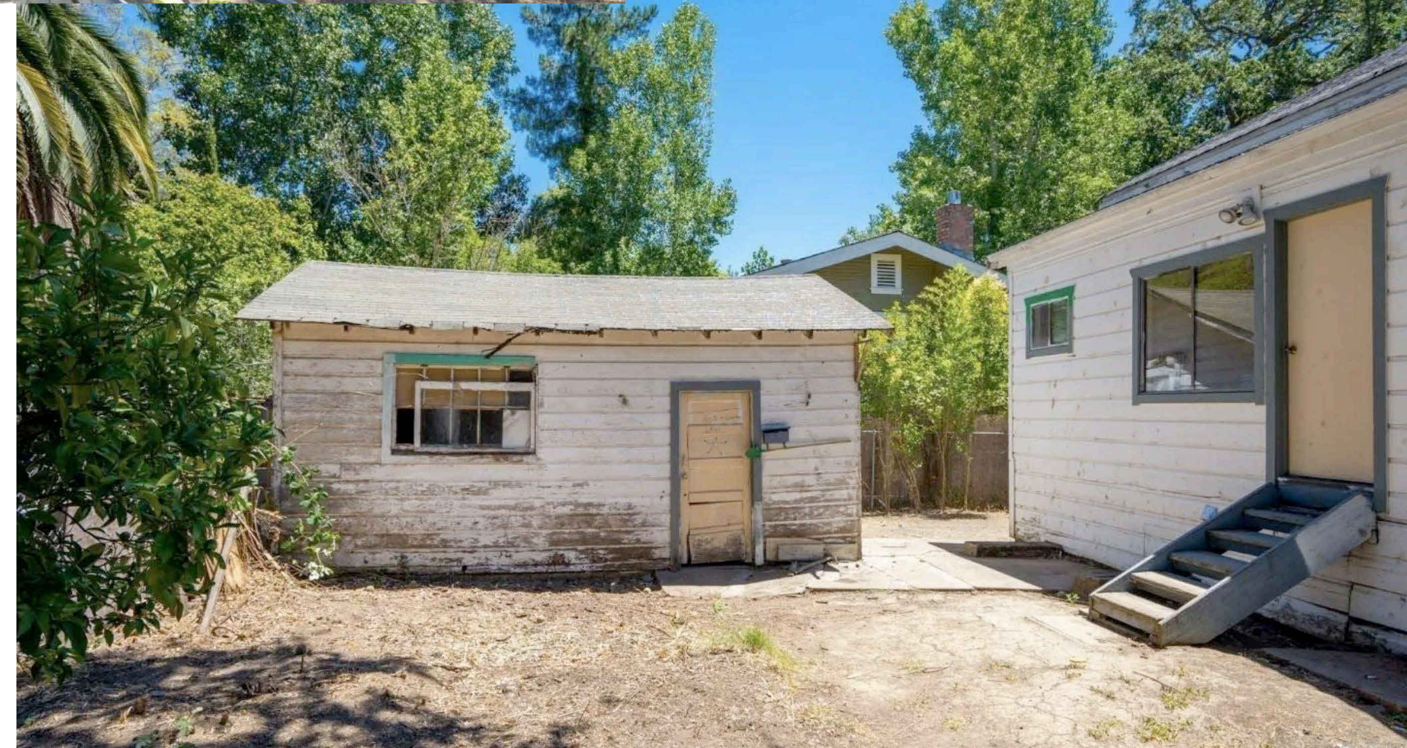
5. Rear Elevation + Garage (Demolished)
