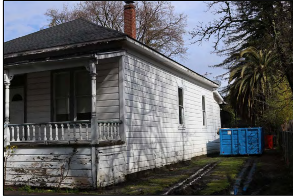
East elevation, SE corner, looking north
