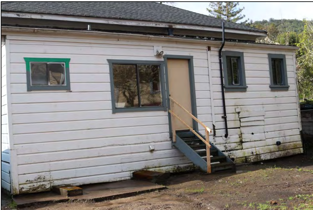
Figure 14: North elevation (rear)
