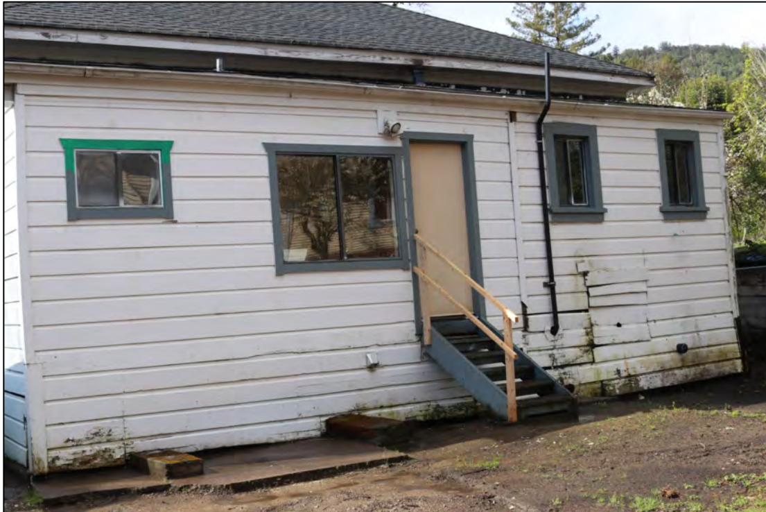
North elevation wing to be modified
