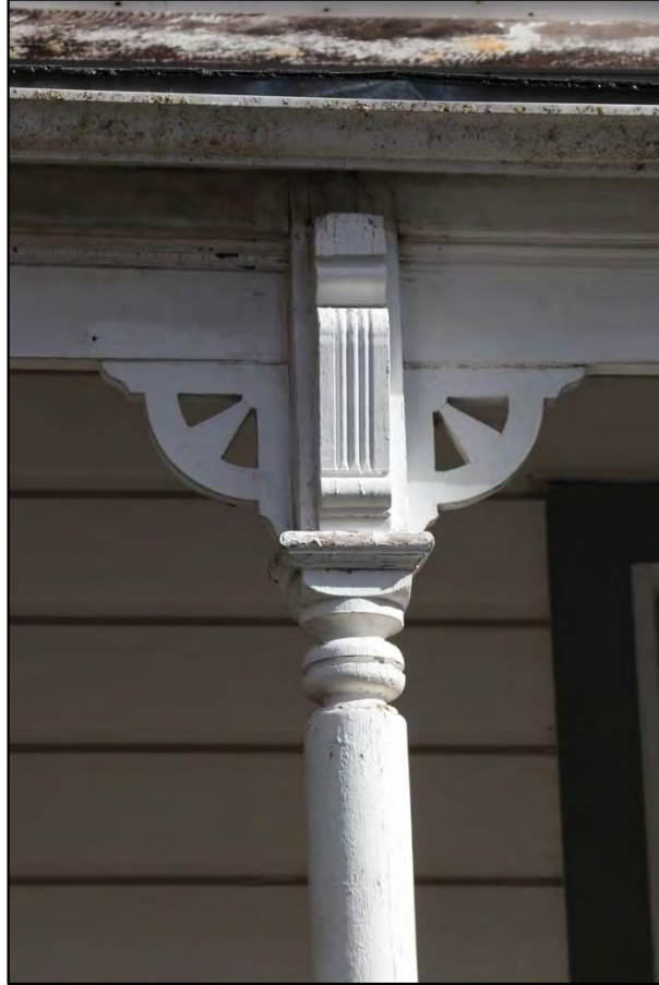
Figure 7: South elevation, bracket on porch post
