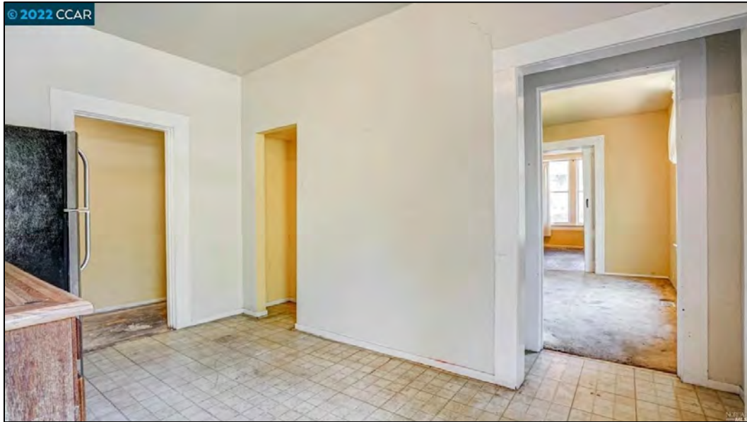
Figure 7: Kitchen, looking SE, door to dining room and opening to hallway
