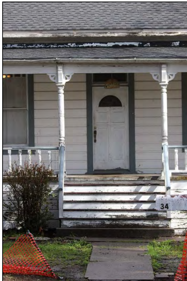
Figure 2: South elevation (front), front door and steps
