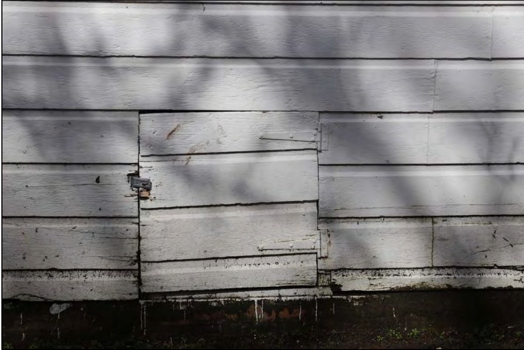
Figure 11: East elevation, foundation access hatch
