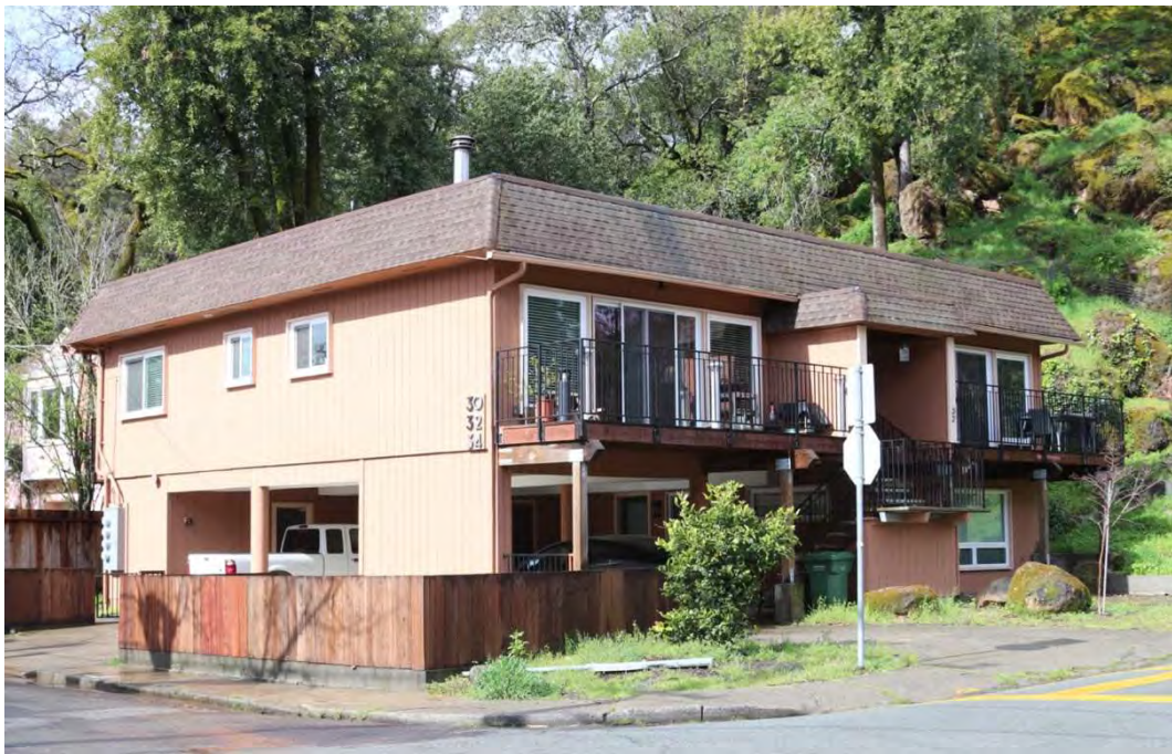
Figure 34: Neighbor on the SW corner of Olema Road and Manor Road
