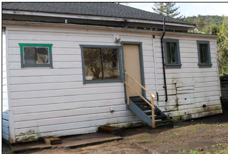
North elevation wing to be modified
