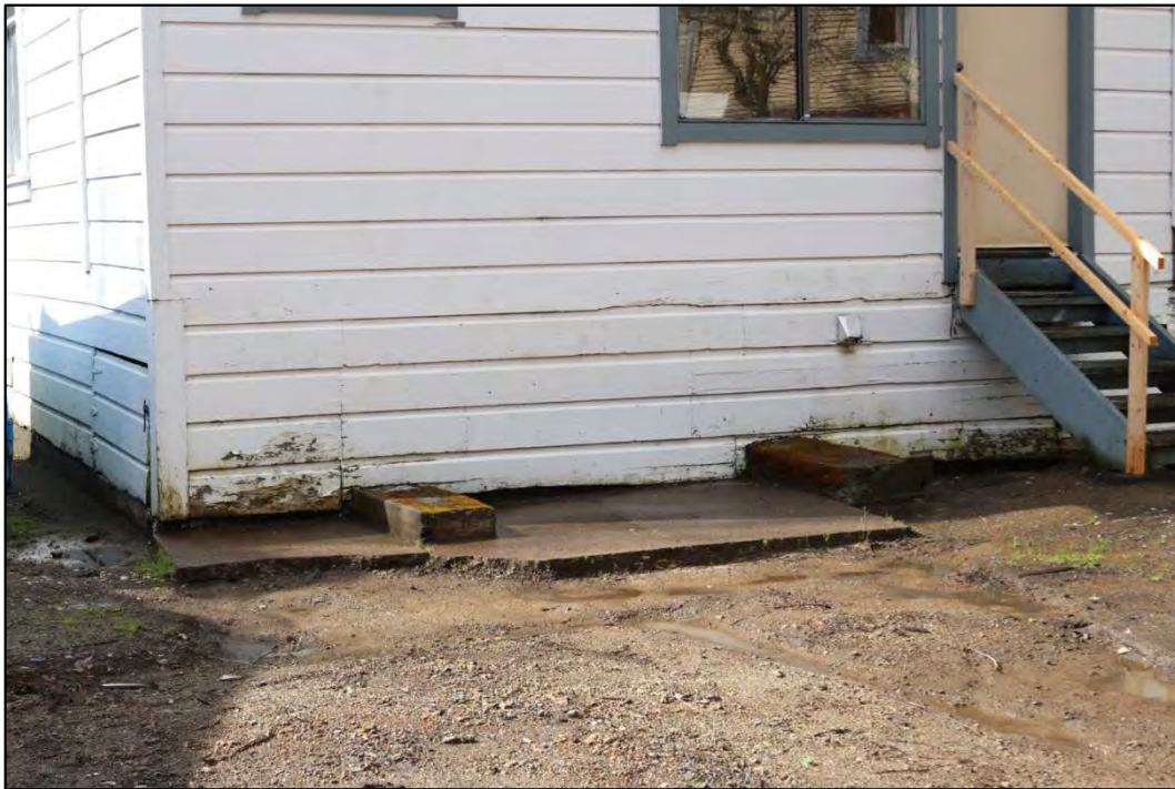
Figure 16: North elevation, foundation of previous porch steps at NE corner
