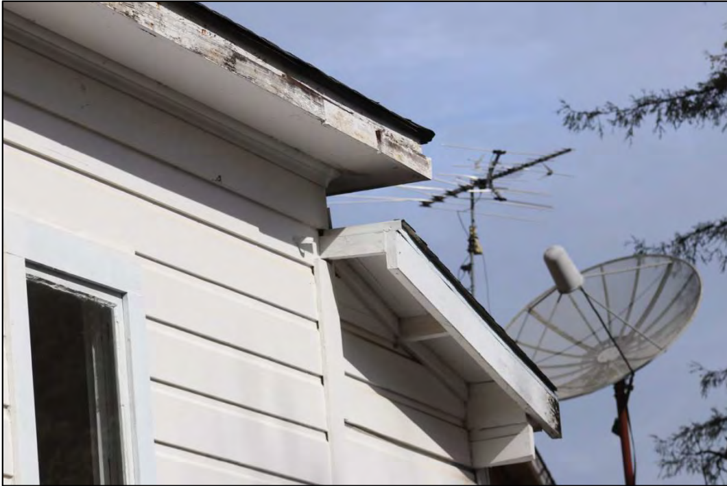
Figure 13: East elevation, NE corner, looking north
