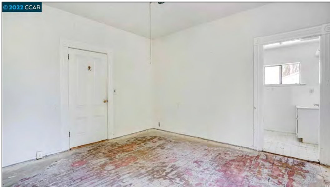
Figure 14: Master bedroom, hall door and opening to master bath
