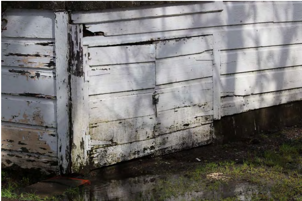
Figure 10: Hatch under front porch at SE corner
