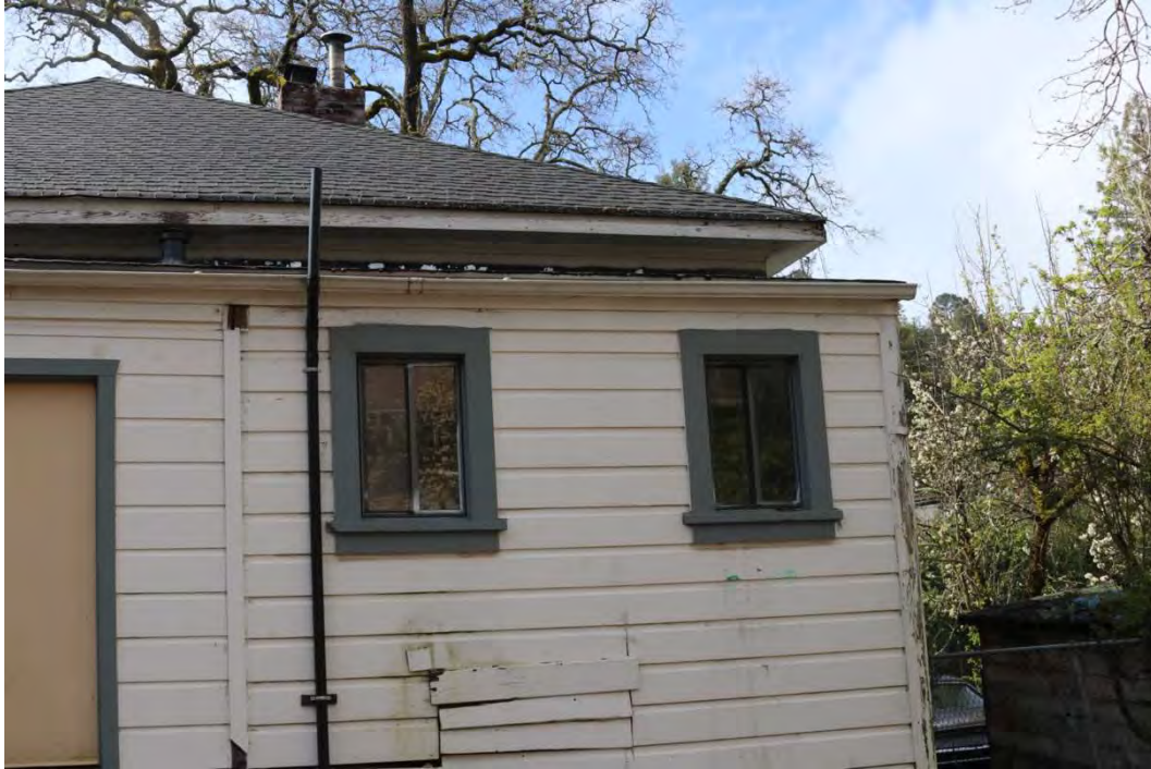
Figure 21: North elevation, modern windows at NW corner
