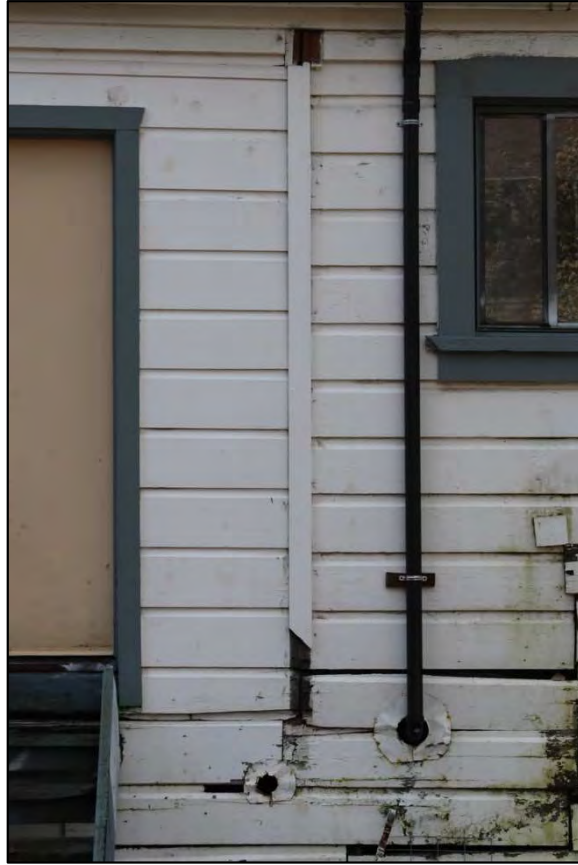
Figure 19: North elevation, junction of infilled porch
