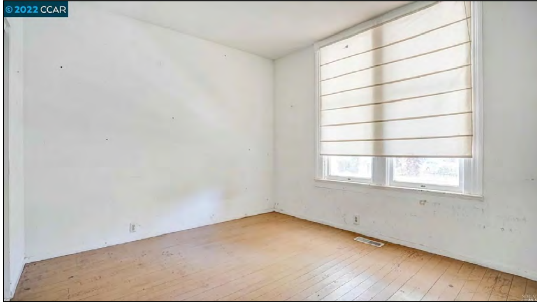
Figure 9: Bedroom #2, looking SE towards front windows
