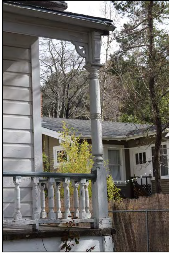
Figure 5: South elevation, SE corner, porch post
