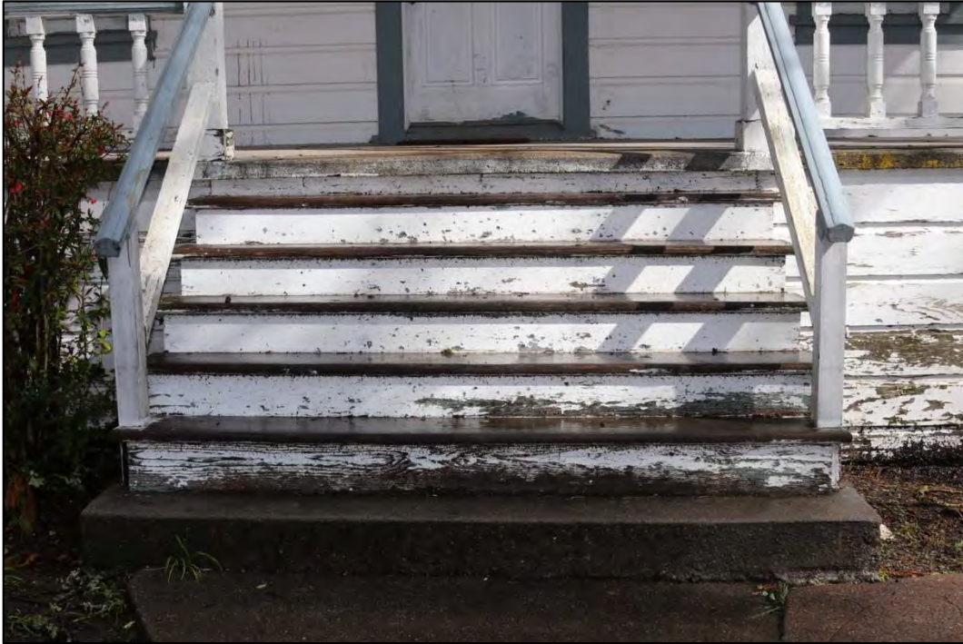
Figure 3: South elevation, front steps
