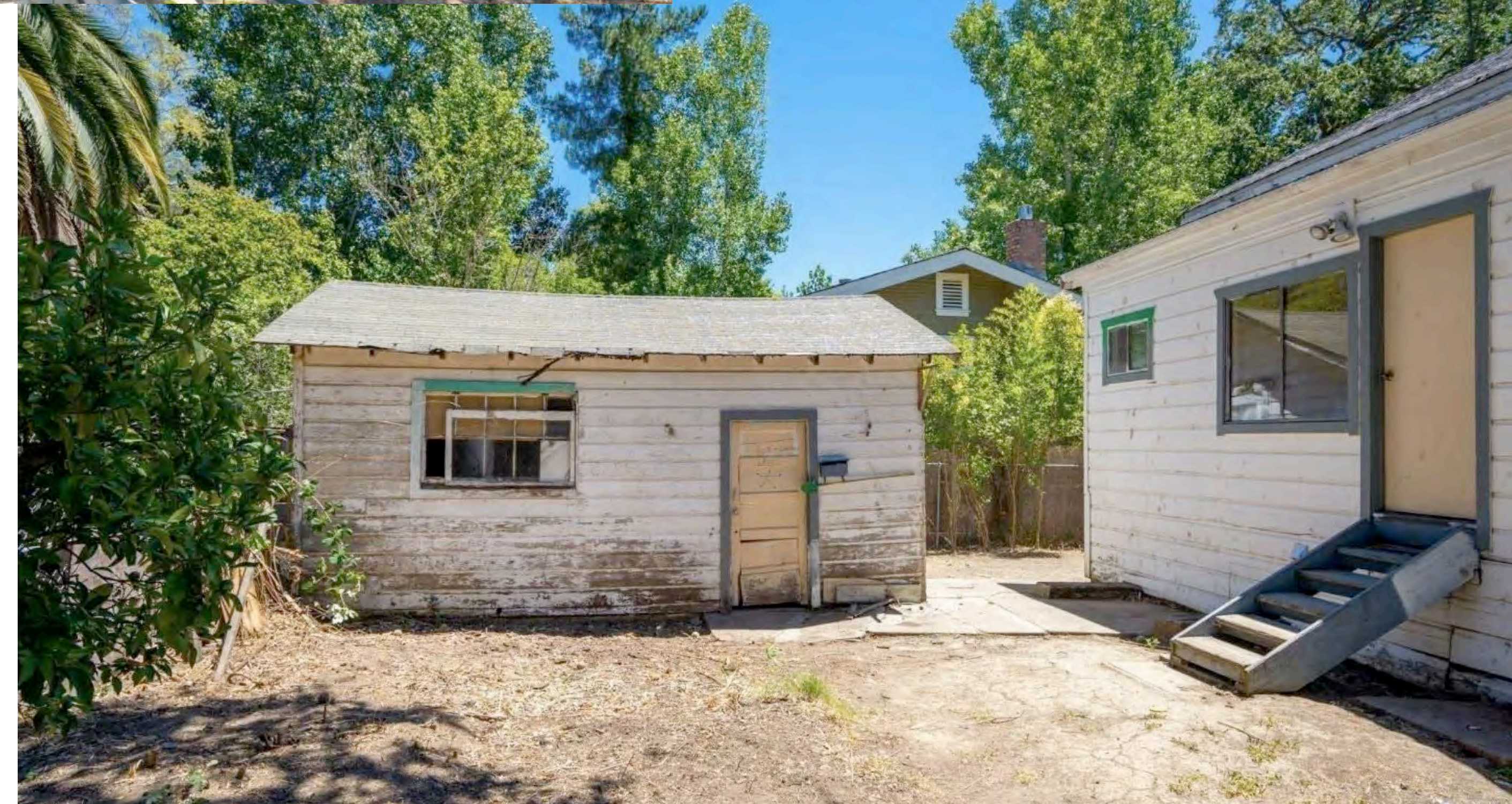
5. Rear Elevation + Garage (Demolished)
