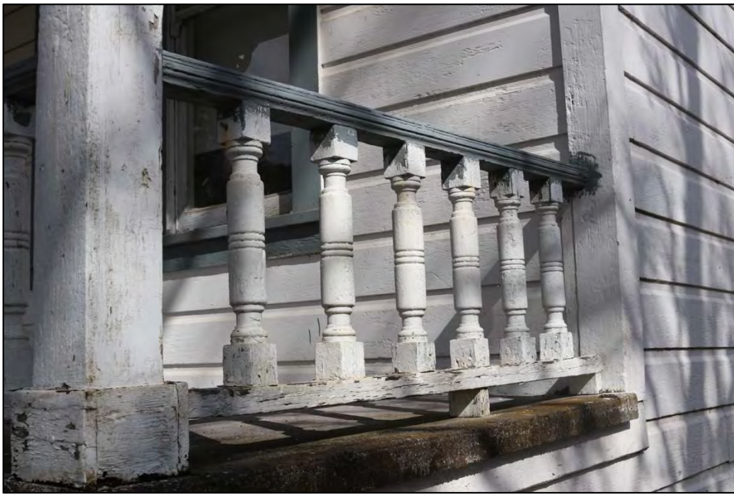
Figure 6: South elevation, porch balustrade
