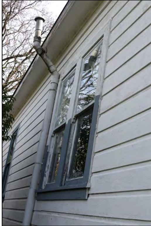
Figure 25: West elevation, pair of windows
