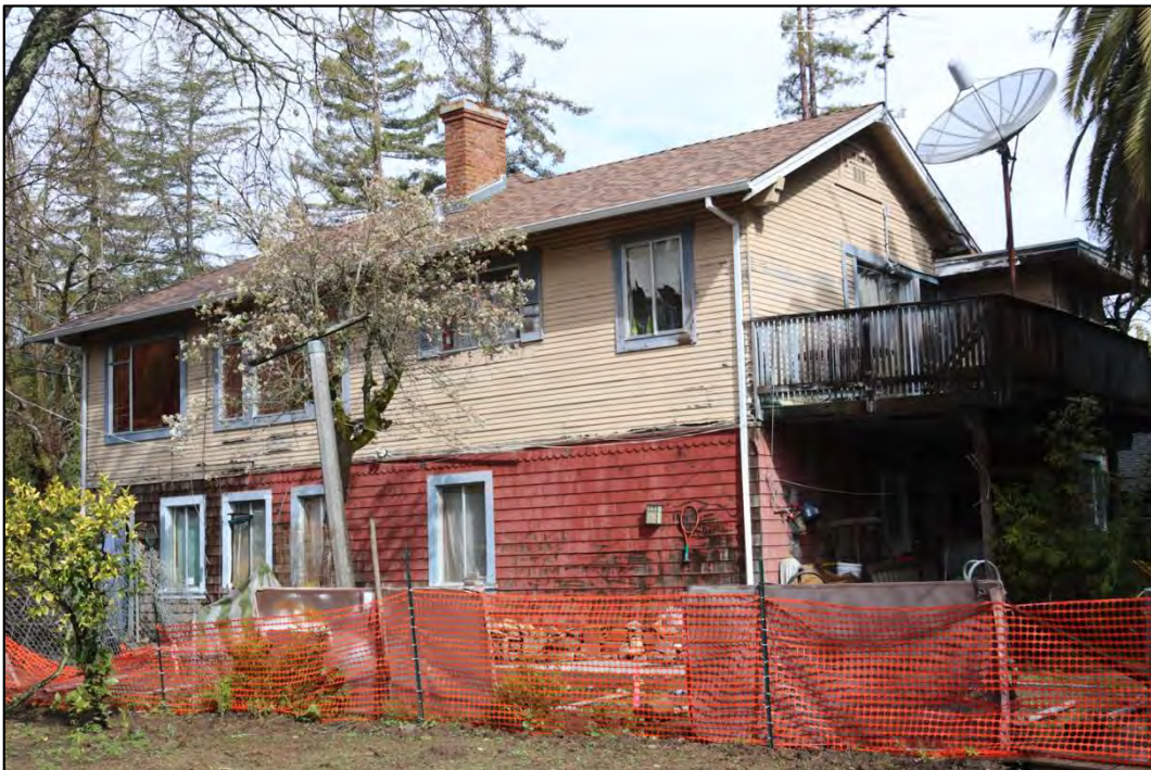
Figure 28: Neighbor to the north as seen from backyard
