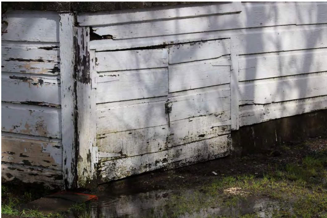
Figure 10: Hatch under front porch at SE corner
