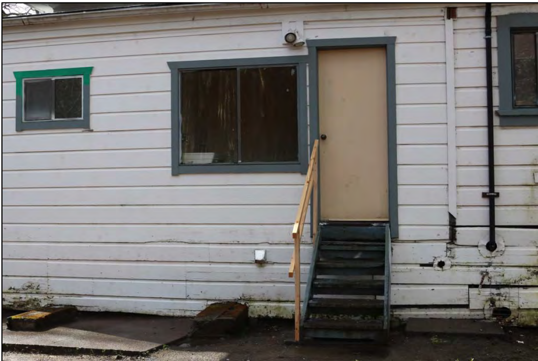
Figure 18: North elevation, back door and steps, modern windows
