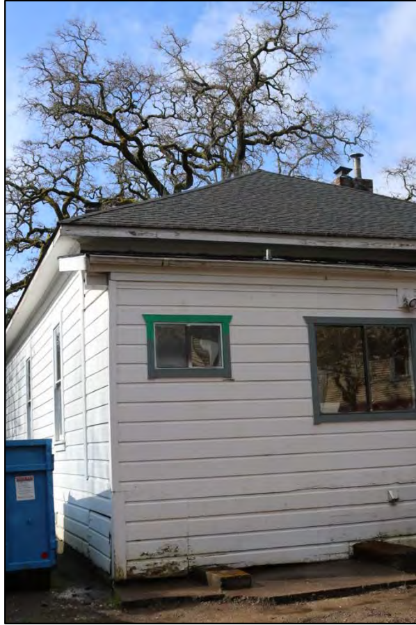
Figure 15: North elevation, modern window at NE corner
