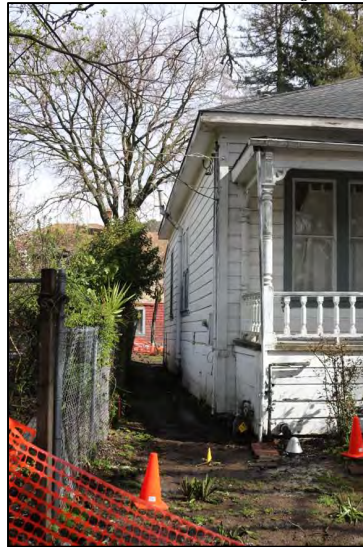
West elevation, looking north
