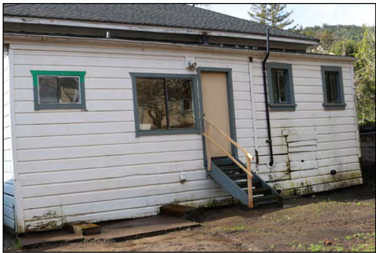
North elevation wing to be modified
