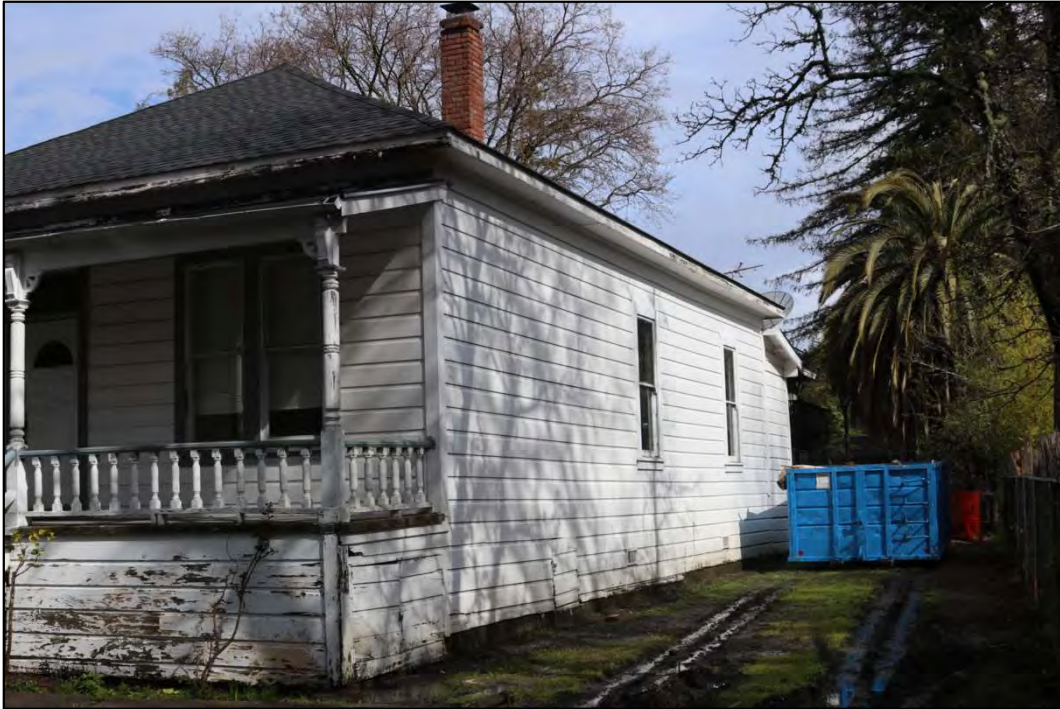
Figure 9: East elevation, looking north
