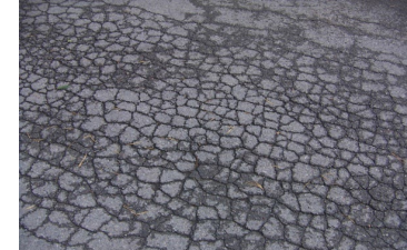
Alligator Cracking
