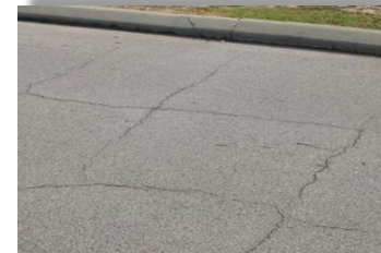
Block Cracking
