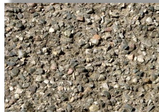
Weathering or Raveling
