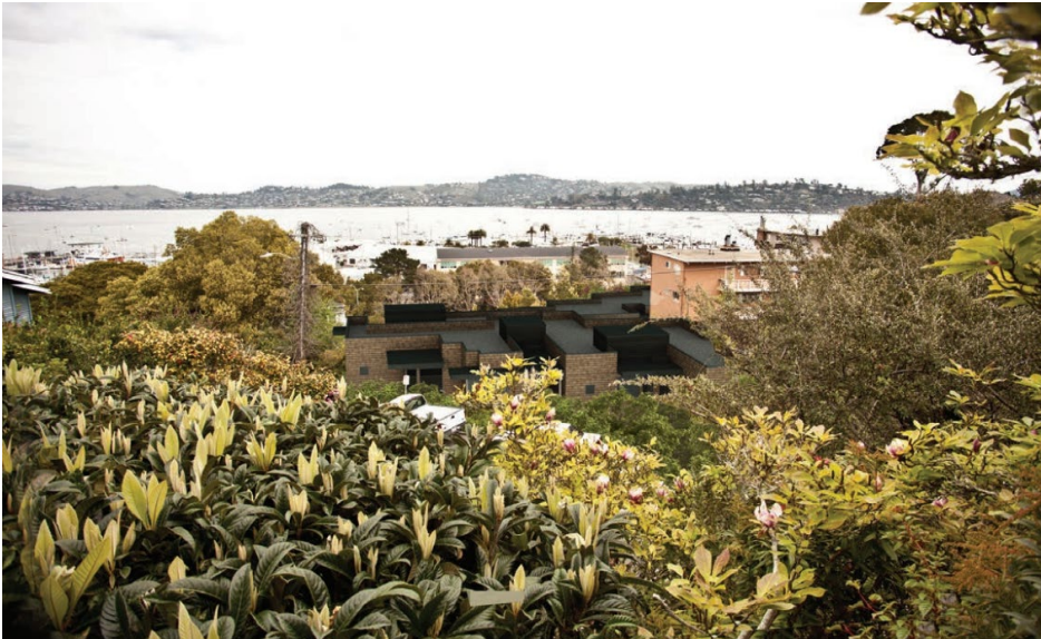
View over Project after Construction
