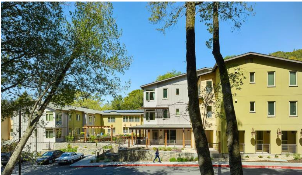
View of Existing Building from Street
