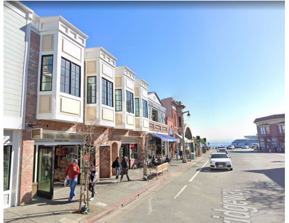
Current Built Conditions after Renovation
