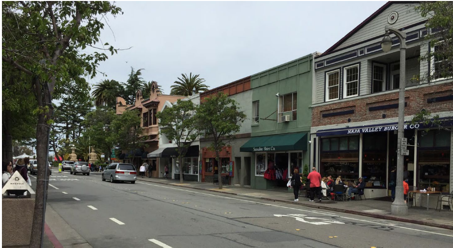
Façade: Before Renovation
