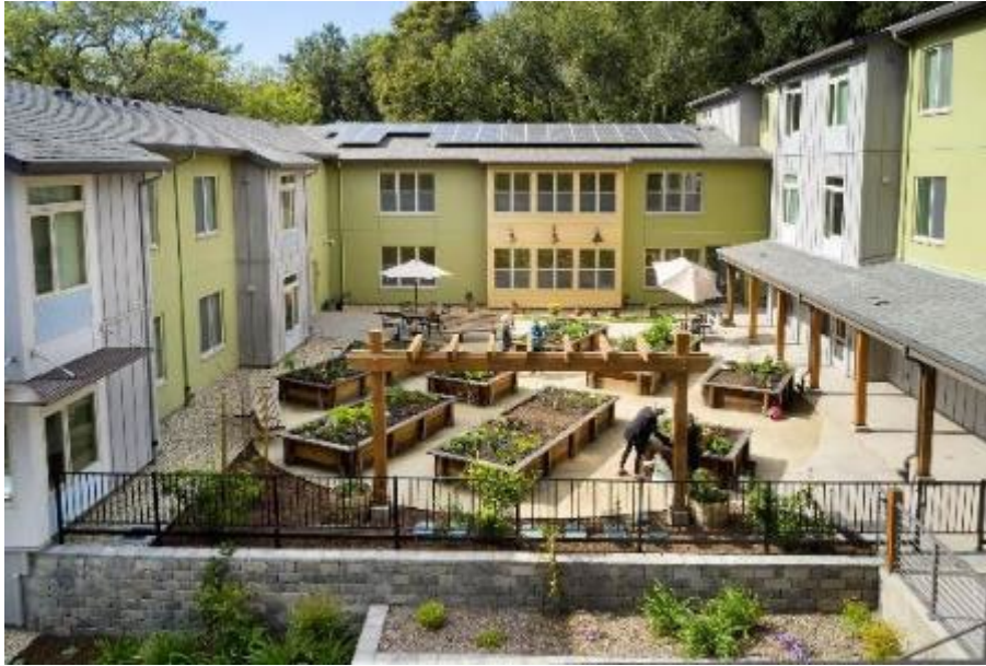
Building Amenity: Courtyard and Garden
