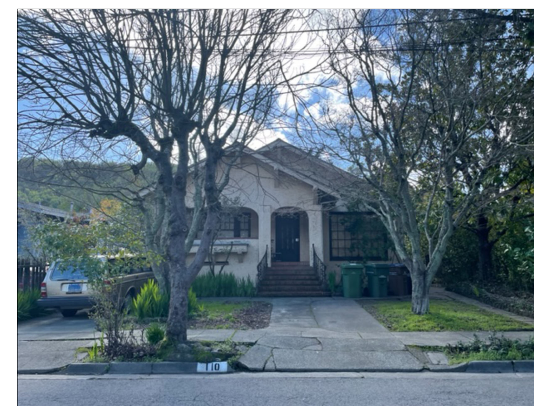
110 MONO AVENUE NEIGHBOR ON LEFT (WEST)
