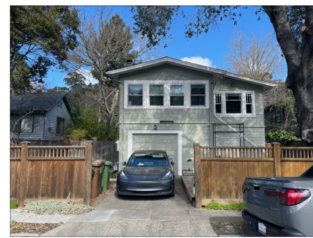
125 MONO AVENUE 2 STORY HOUSE ACROSS STREET
