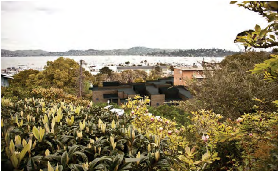
View over Project after Construction
