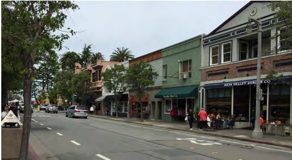
Façade: Before Renovation
