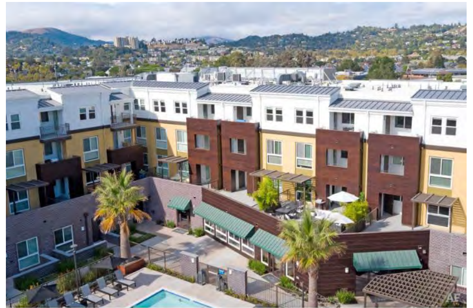
Bird's Eye View of Building
