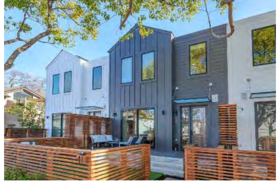
Backyards of Built Property
