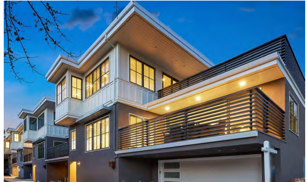
Newly Built Building
