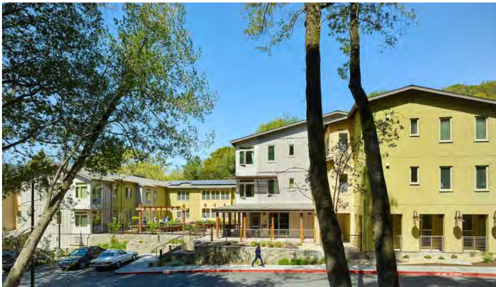
View of Existing Building from Street
