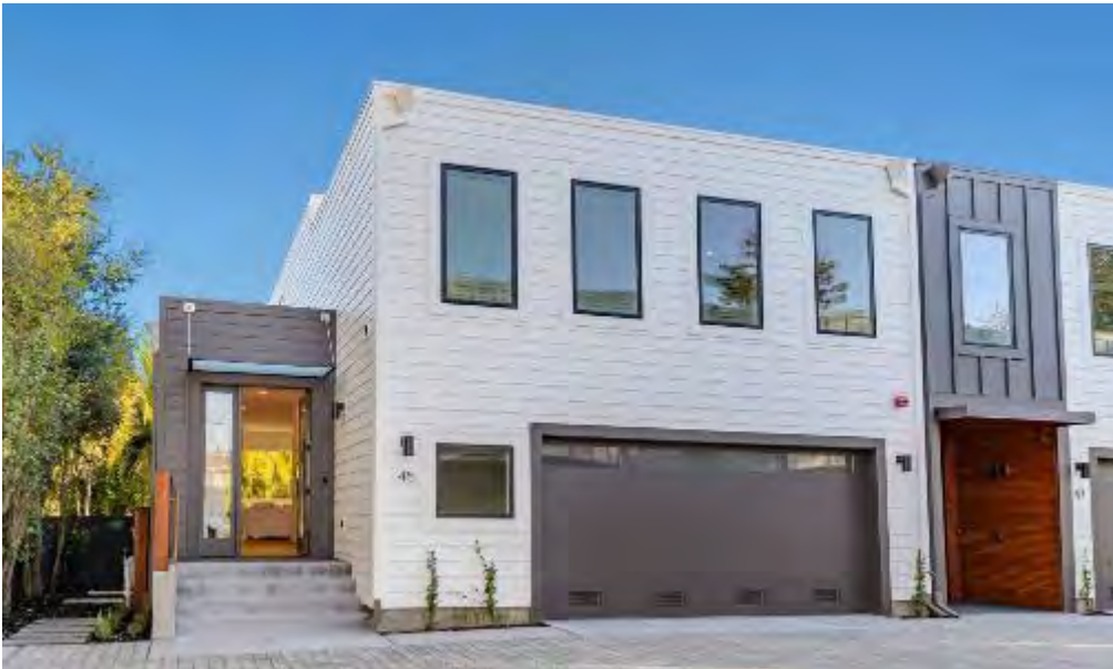
Newly Built Building
