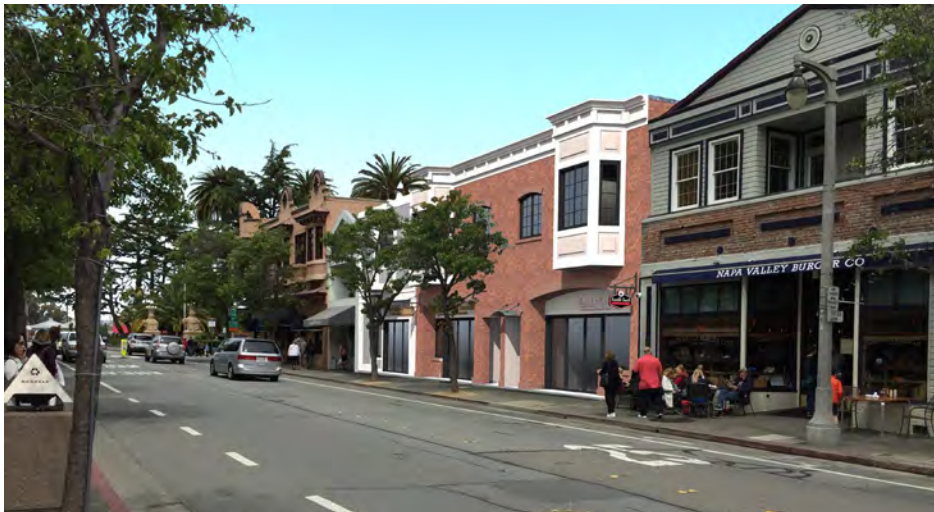
Façade: After Renovation
