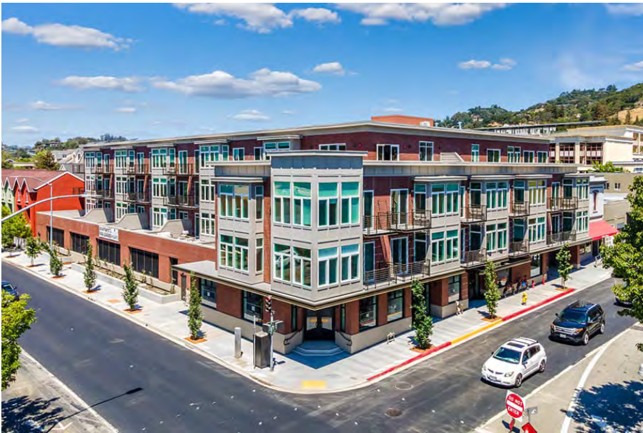
Existing Building Facade
