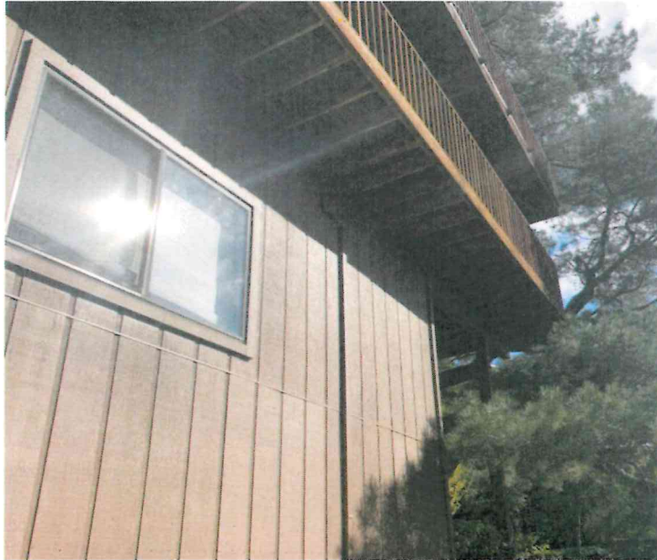
Figure 6. Ground Floor Western Wall to Be Demolished
