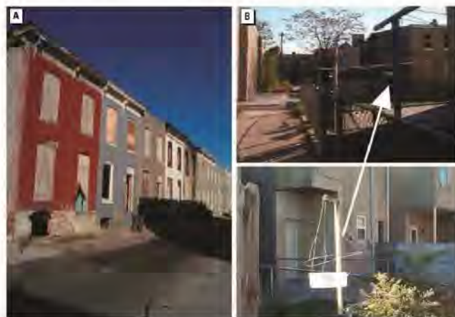
Figure 2. Before demolition, site 1. (A) Row houses. (B) Dust-fall collection apparatus with arrow pointing to another view of the same sampling location.
