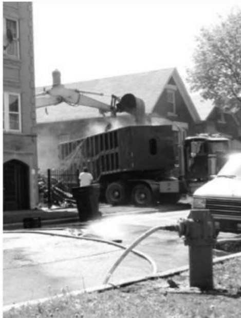
Photo 4. Limited dust suppression in use at a Chicago demolition site. Source: University of Illinois at Chicago
