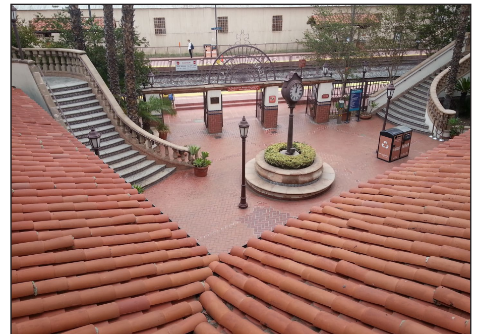
Photo 6. View of the courtyard at the Santa Ana Regional Transit Center.
