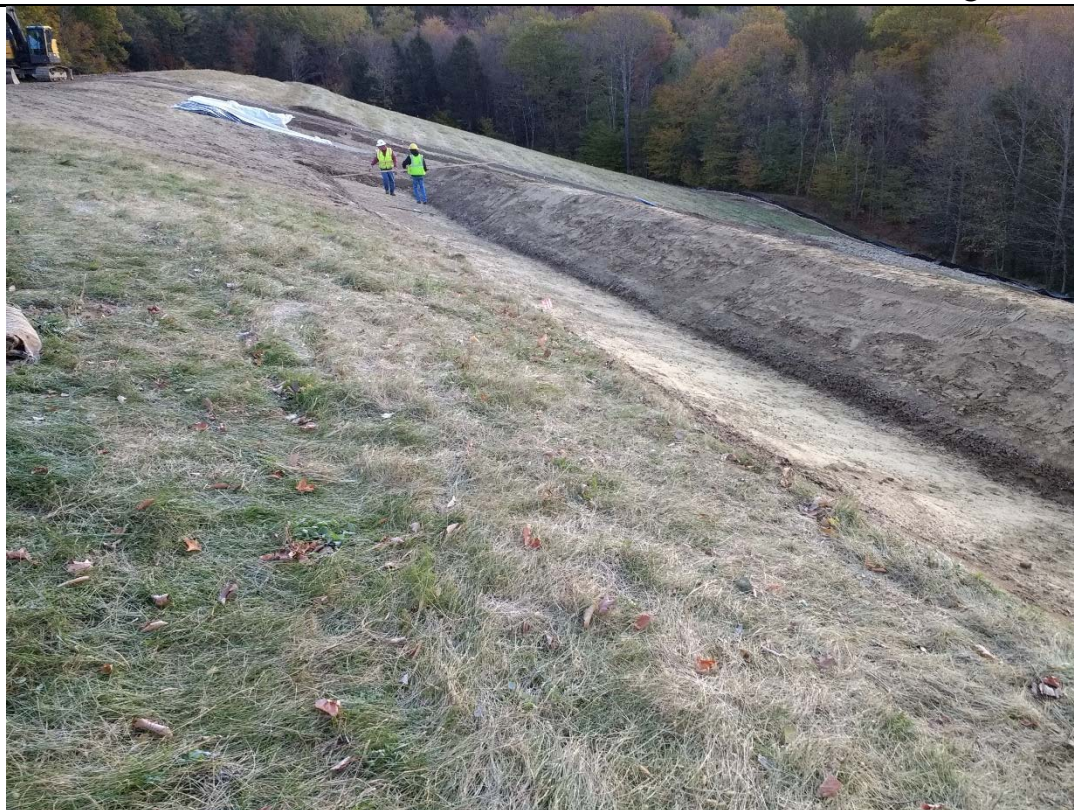
10/26/18: Construction of diversion berm, west of downslope swale at intersection with downslope swale
