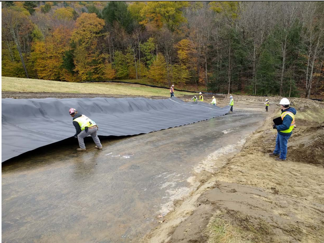
10/31/18: Installation of 60-mil channel liner in downslope swale
