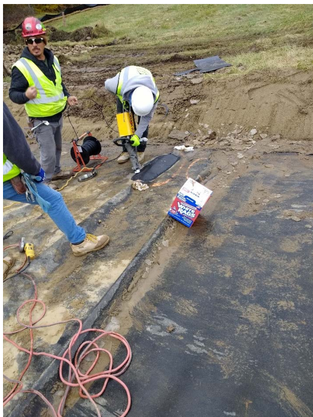
10/31/18: Extrusion welded patch repairs to existing cap
