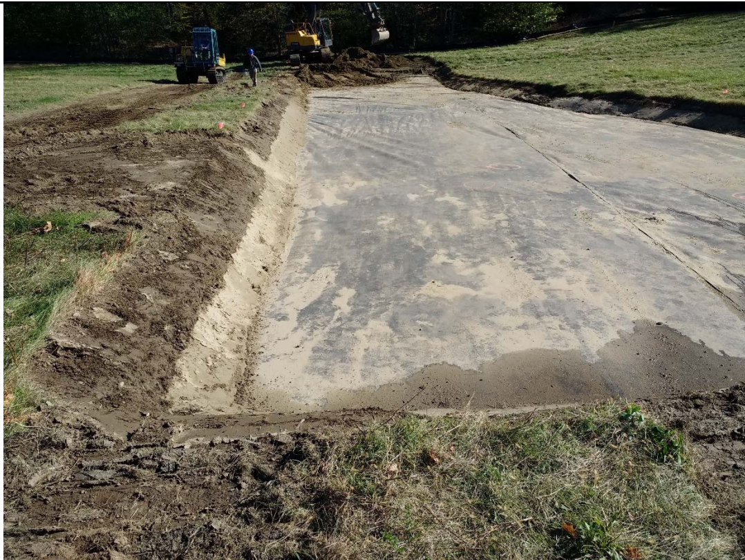
10/18/18: Removal of cap soils within limits of downslope swale
