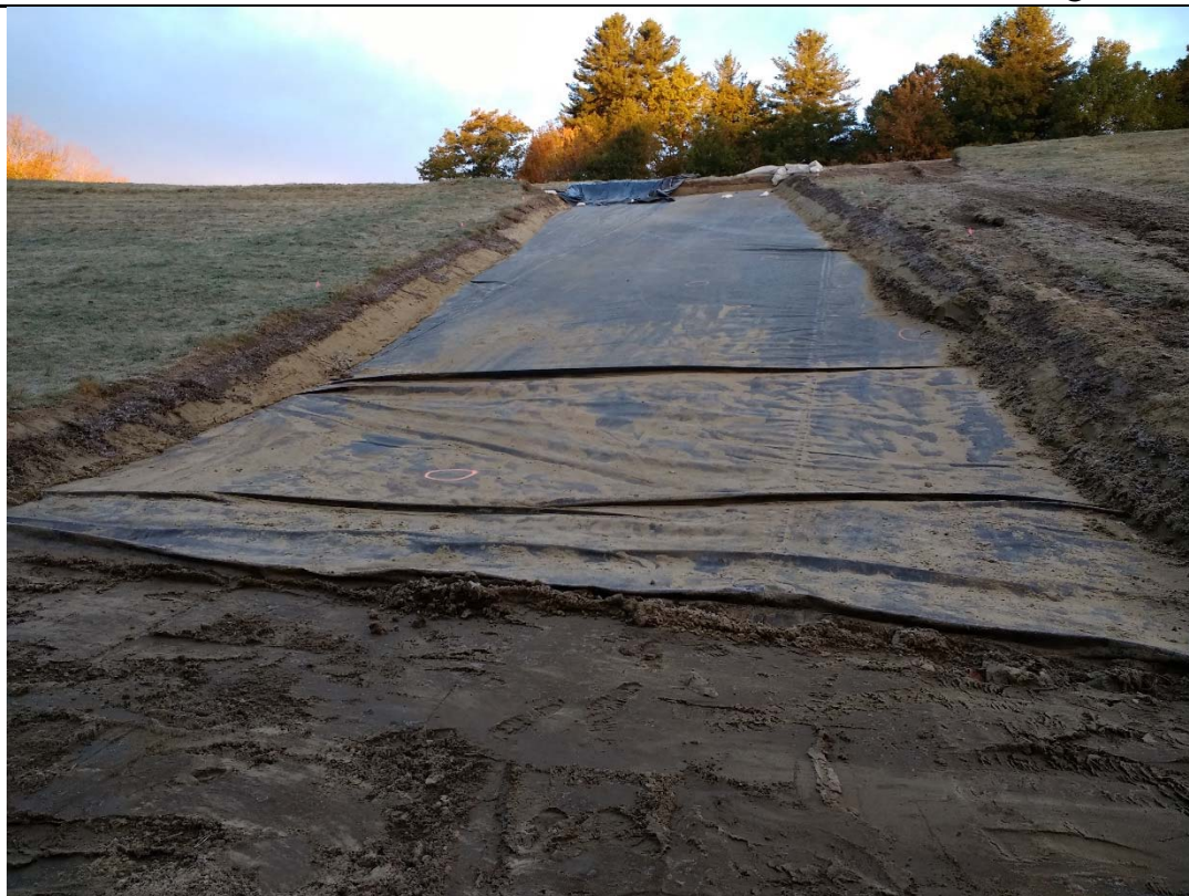
10/22/18: Completed removal of cap soils within downslope swale
