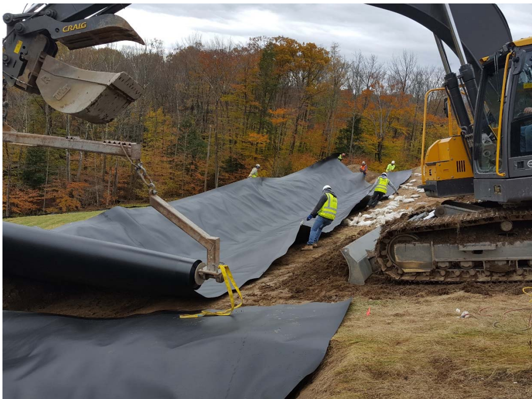
10/31/18: Installation of 60-mil channel liner in diversion berm west of downslope swale
