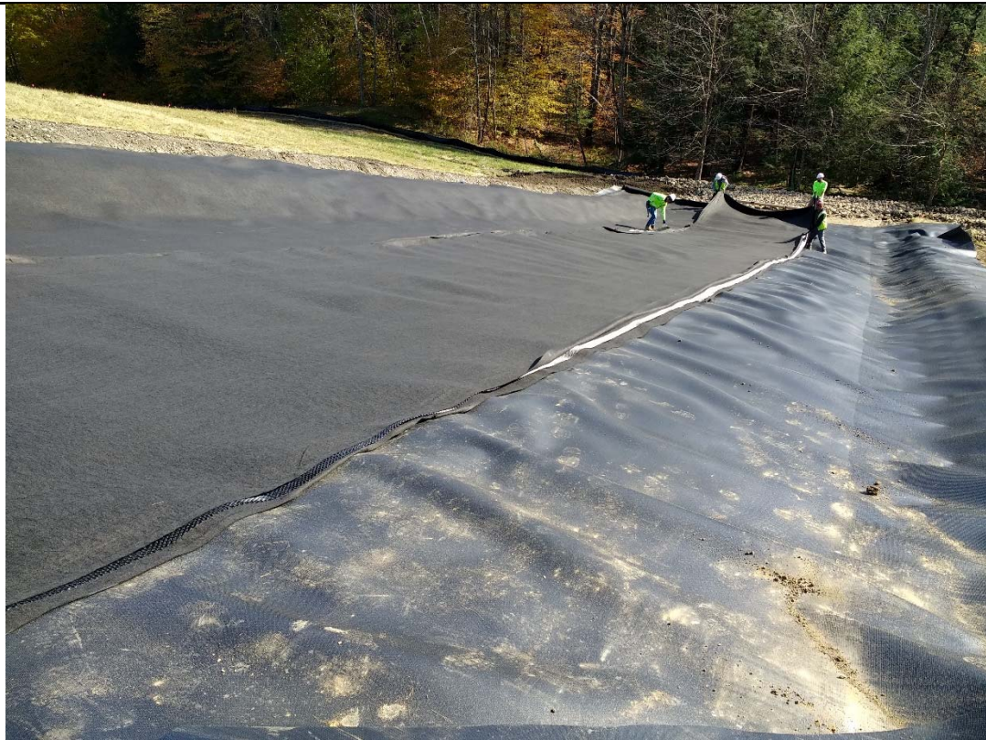
10/31/18: Installation of 250-mil geocomposite in downslope swale
