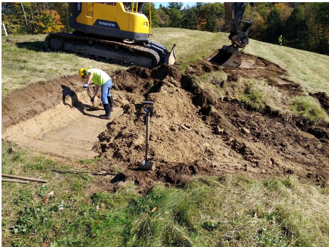
10/17/18: Removal of cap soils within limits of downslope swale
