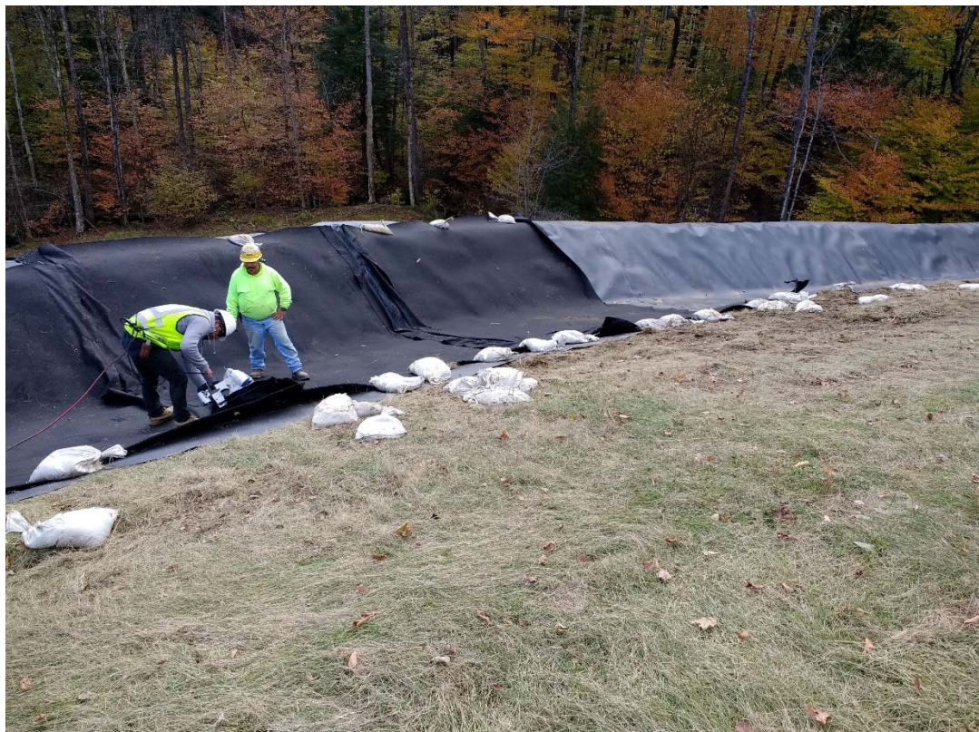
10/31/18: Installation of 250-mil geocomposite in diversion berm west of downslope swale
