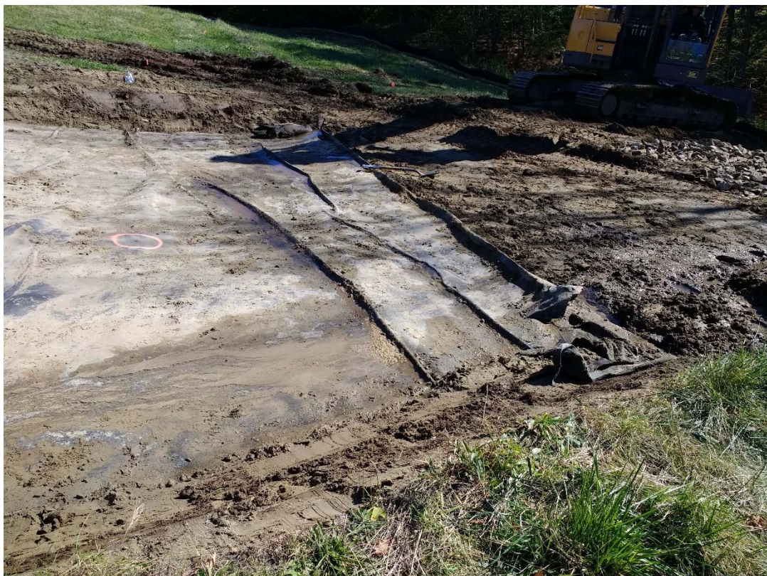
10/18/18: Existing wrinkles in the existing 40-mil cap at toe of slope of proposed downslope swale
