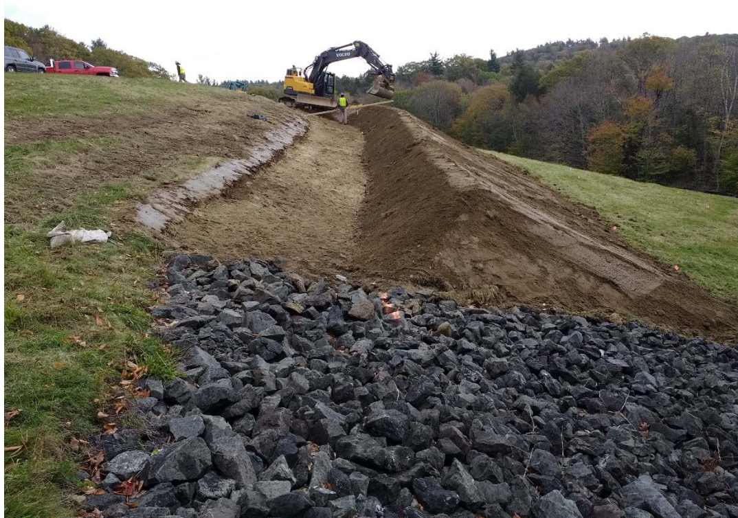
10/23/18: Construction of diversion berm, west of downslope swale at intersection with existing splash pad
