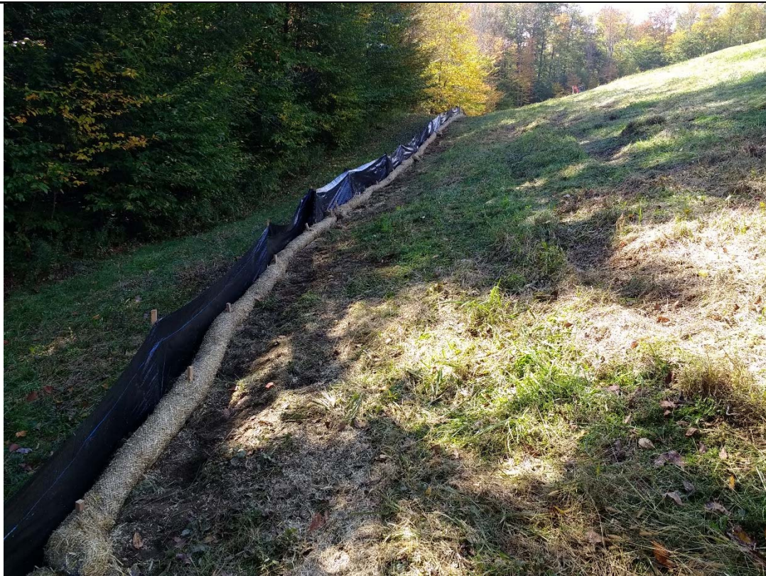
10/10/18: Installation of erosion control measures
