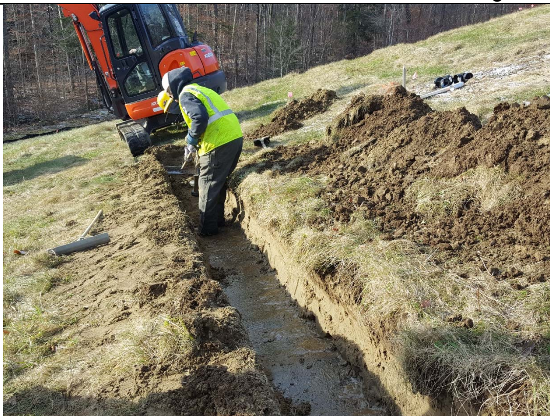
11/14/18: Trench excavation for sub drain piping
