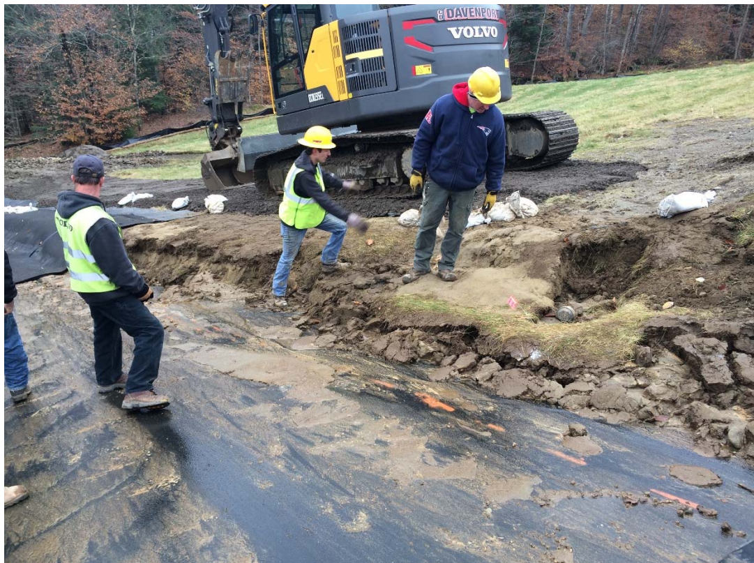
11/5/18: : Side slope of landfill cap in down slope swale following rain event.
