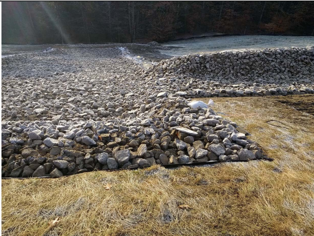
11/9/18: Down slope swale and diversion berm following placement of stone
