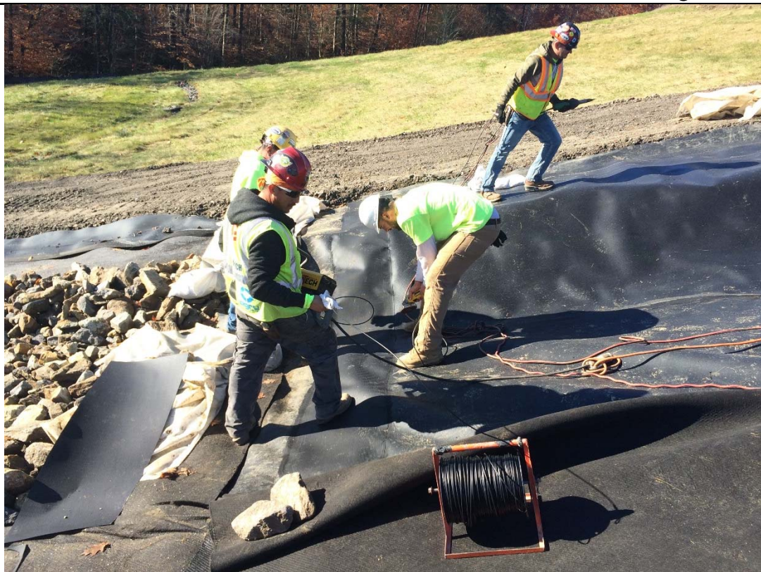
11/7/18: Repairs to channel liner in down slope swale
