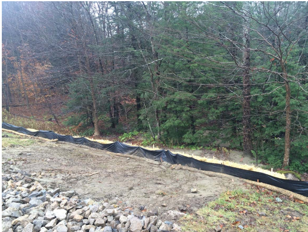
11/6/18: Repaired toe of slope and erosion control barriers at bottom of down slope swale
