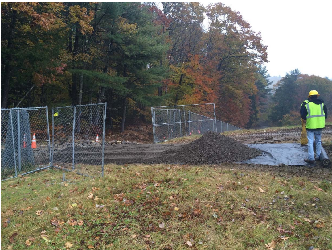
11/1/18: Extension of temporary access road at equipment access gate
