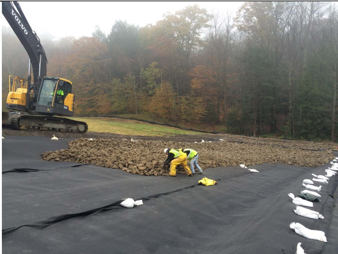
11/1/18: Placement of stone down slope swale
