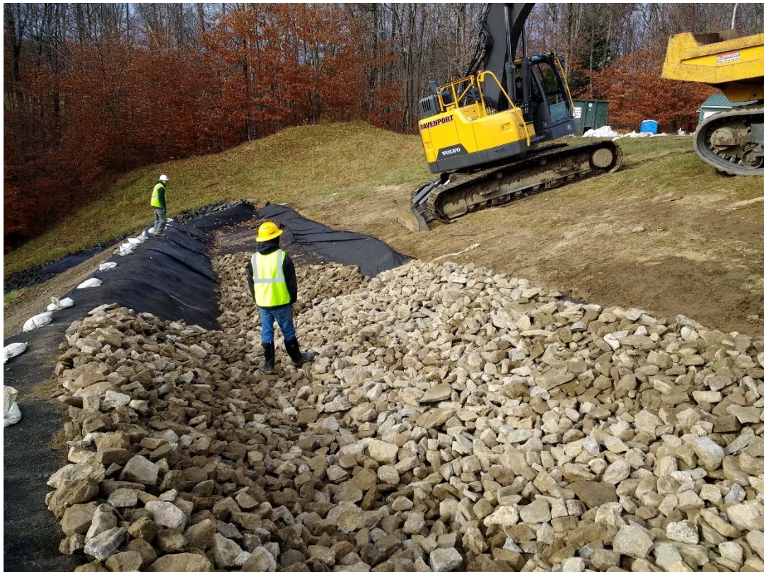
11/9/18: Placement of stone in diversion berm following repairs to channel liners
