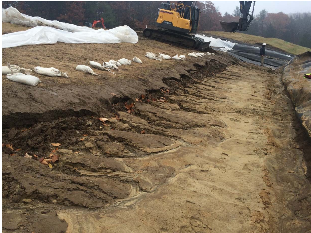
11/6/18: Side slope of landfill and bottom of diversion berm following rain event and removal of channel liner and geocomposite
