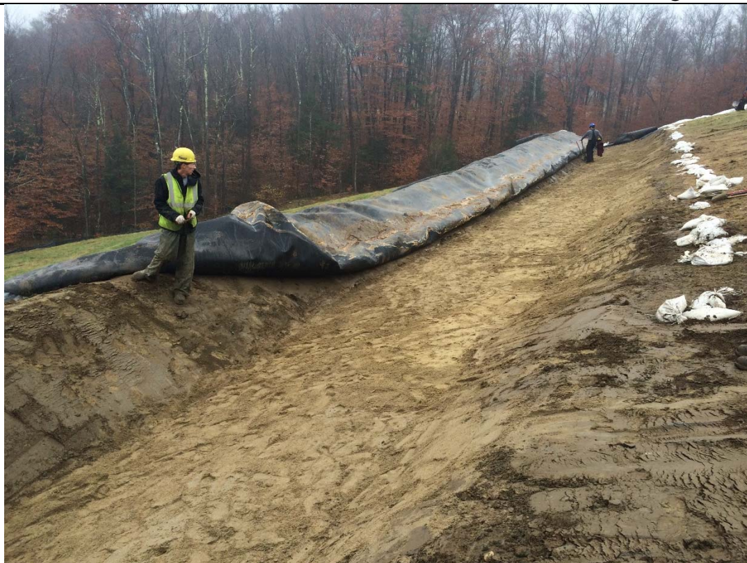
11/6/18: Diversion berm following removal of eroded materials and repair of drainage sand layer and side slope
