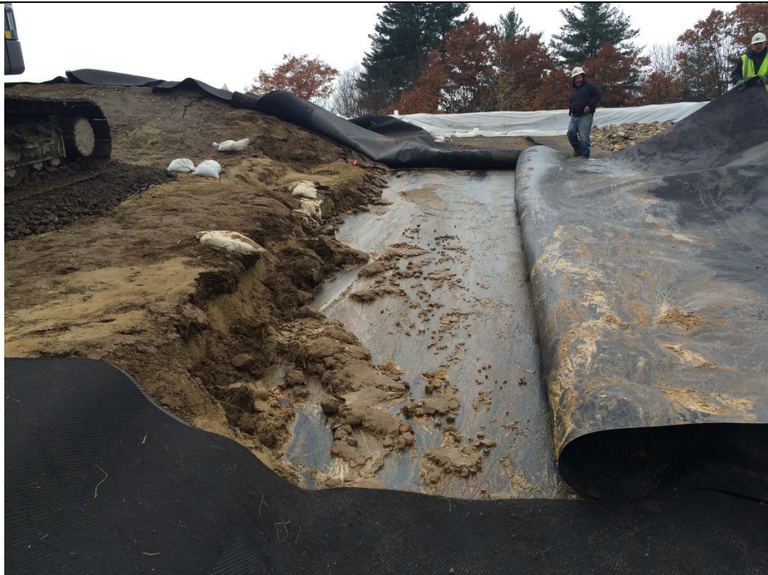
11/5/18: Erosion in down slope swale following rain event. Down slope channel liner and geocomposite has been cut and folded back.
