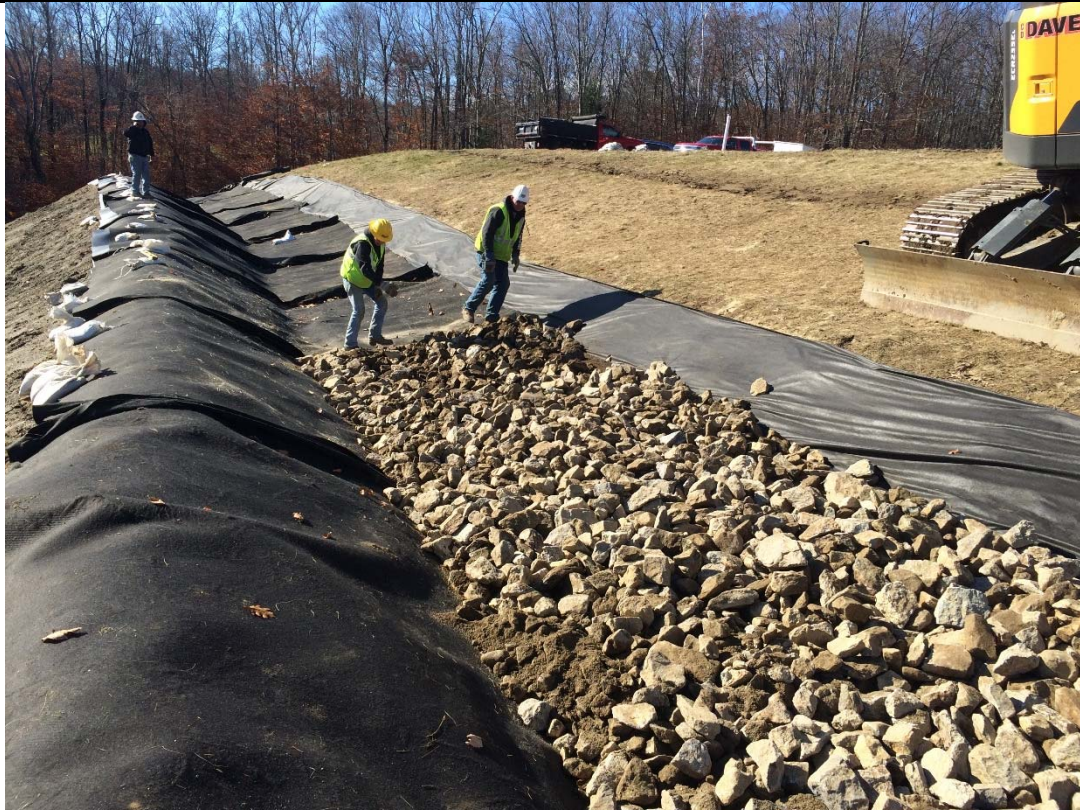
11/8/18: Placement of stone in diversion berm following repairs to channel liners
