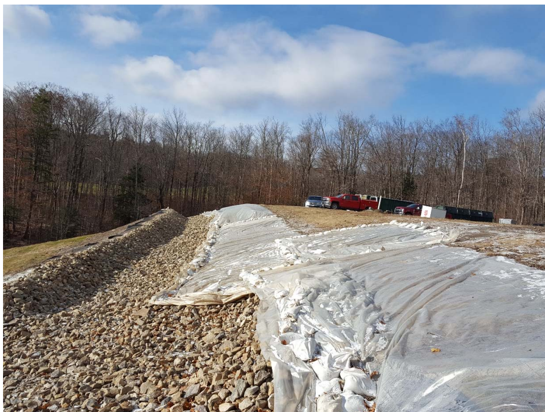
11/14/18: Plastic sheets above diversion berm and down slope swale following placement of stone
