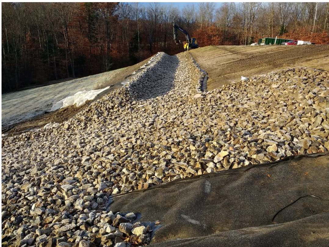
11/9/18: Diversion berm and down slope swale following placement of stone
