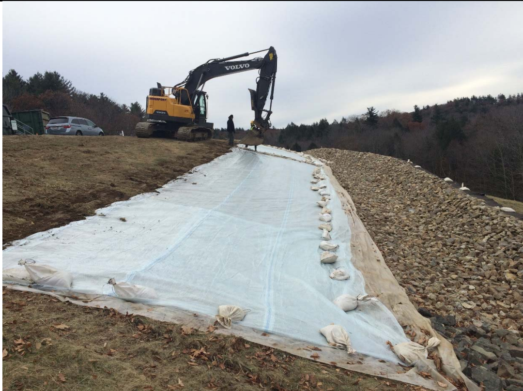
11/15/18: Plastic sheets above diversion berm following placement of stone
