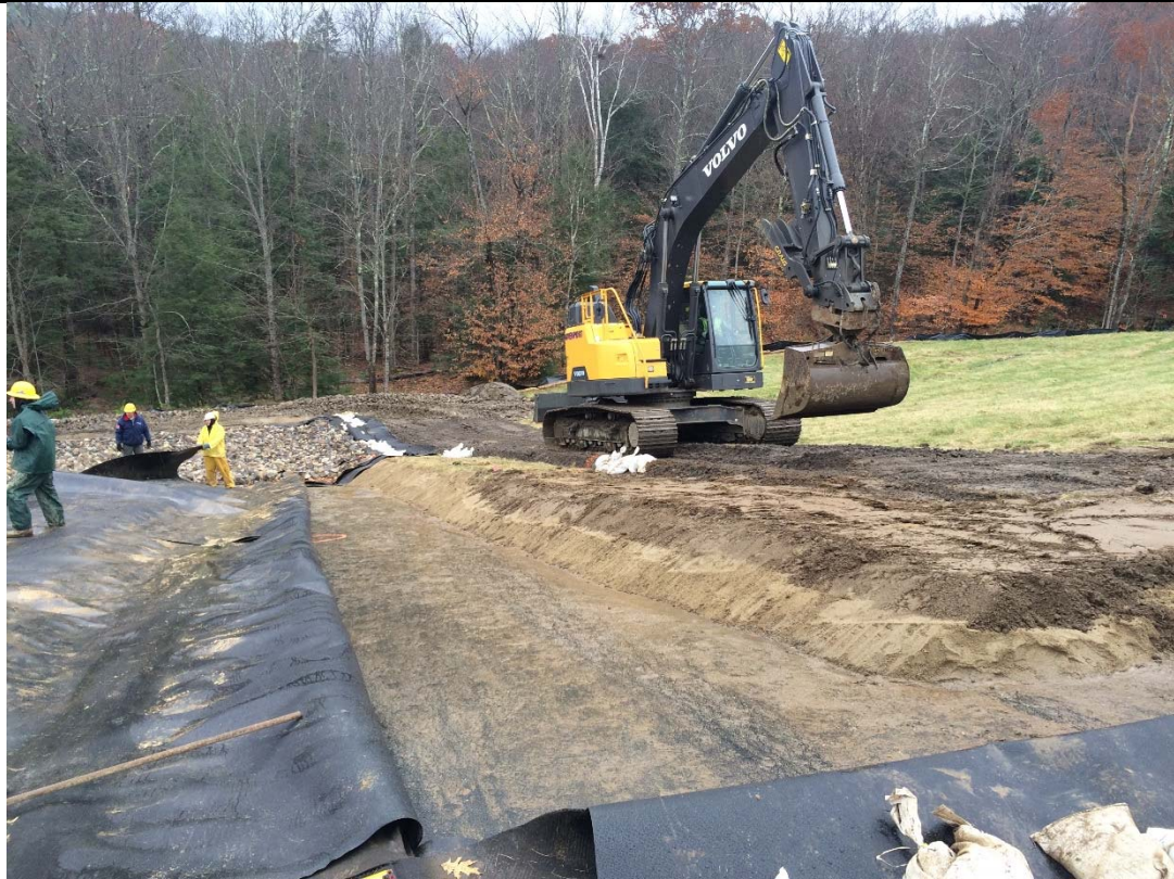
11/5/18: Side slope of landfill cap in down slope swale following removal of eroded materials and repair to side slope.
