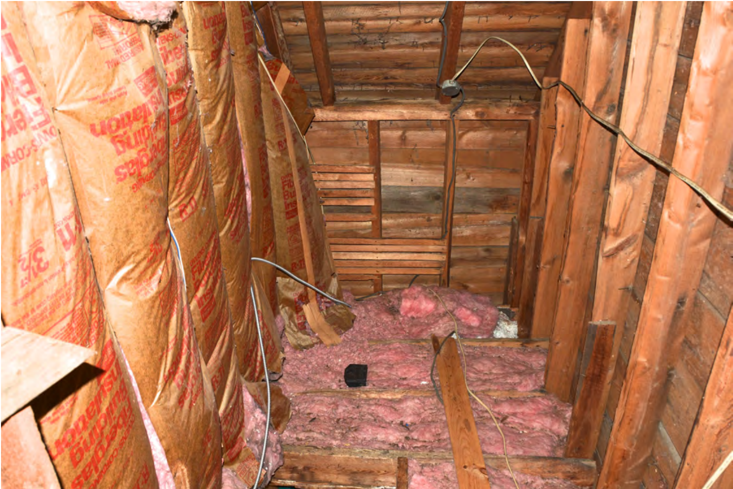
This is a picture of the ceiling area above the closet in the northeast corner of the building.
