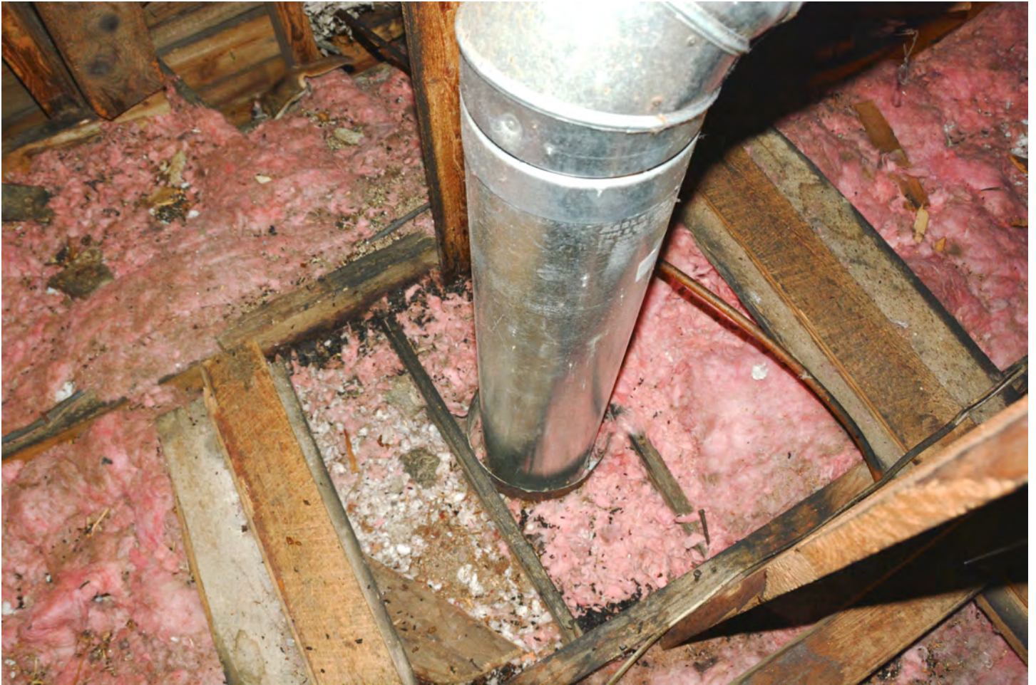
This is the vent pipe for the propane heater that's in the ceiling of the Museum. My main concern here is whether or not there is an appropriate separation between the exhaust pipe and the wooden framing around it. I will follow up with the Building Inspector to seek his opinion.
