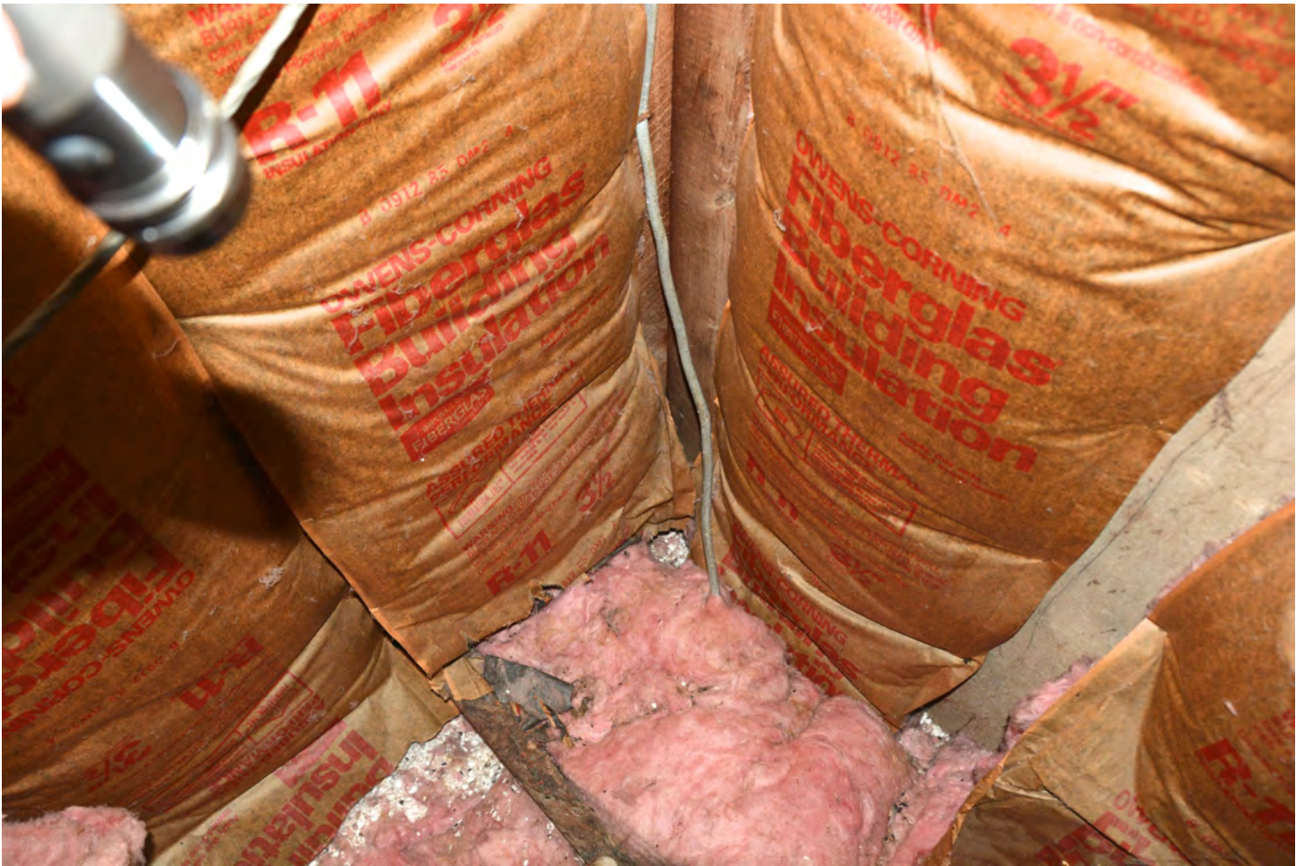
This is a corner of the ceiling above the closet. Note the mouse hole in the insulation in the center of the picture.
