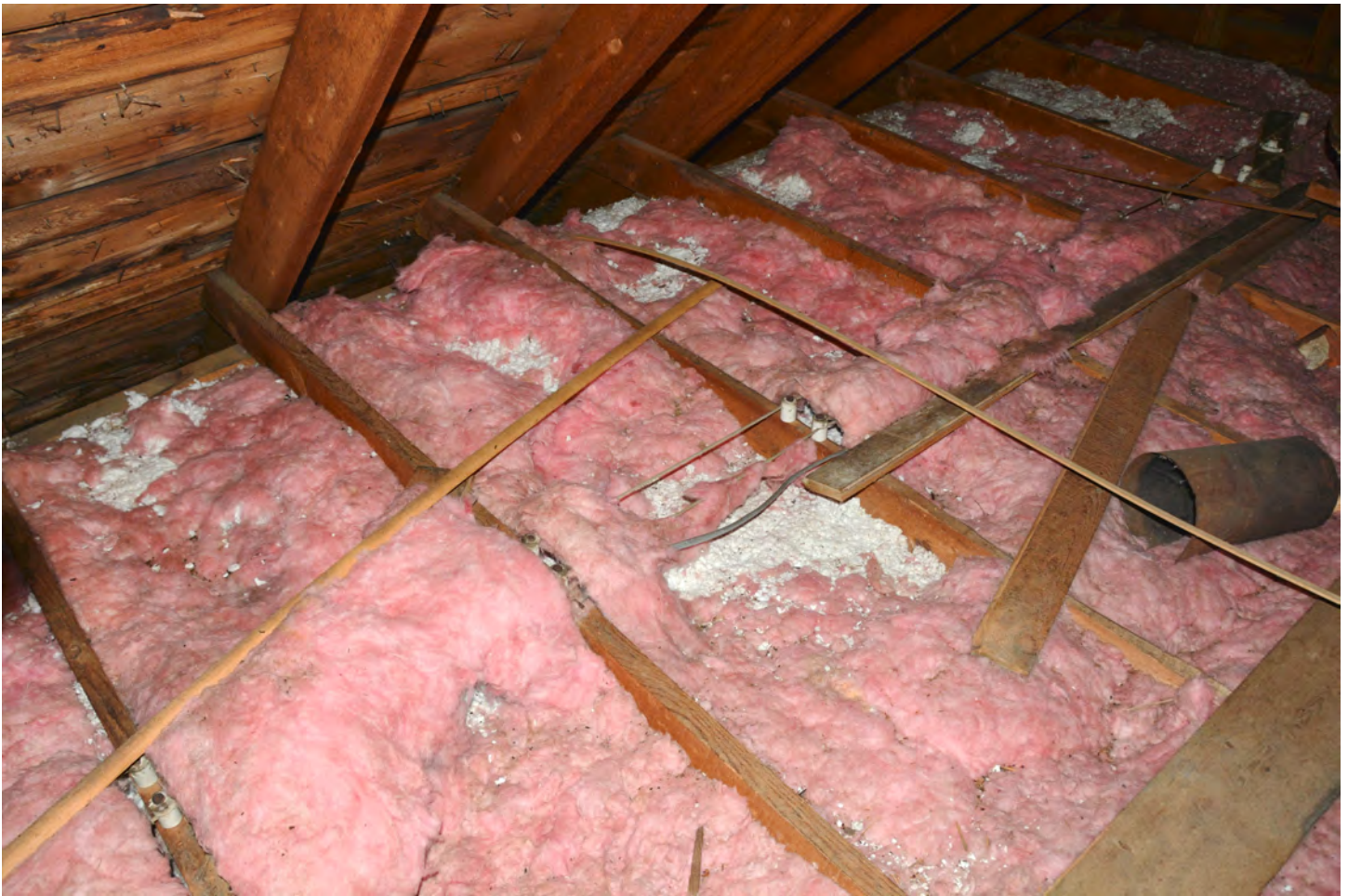
In this picture, you can see how the mice have eaten away at the insulation that was placed on top of the electrical wires and exposing the white insulation (blown in?) below it.
