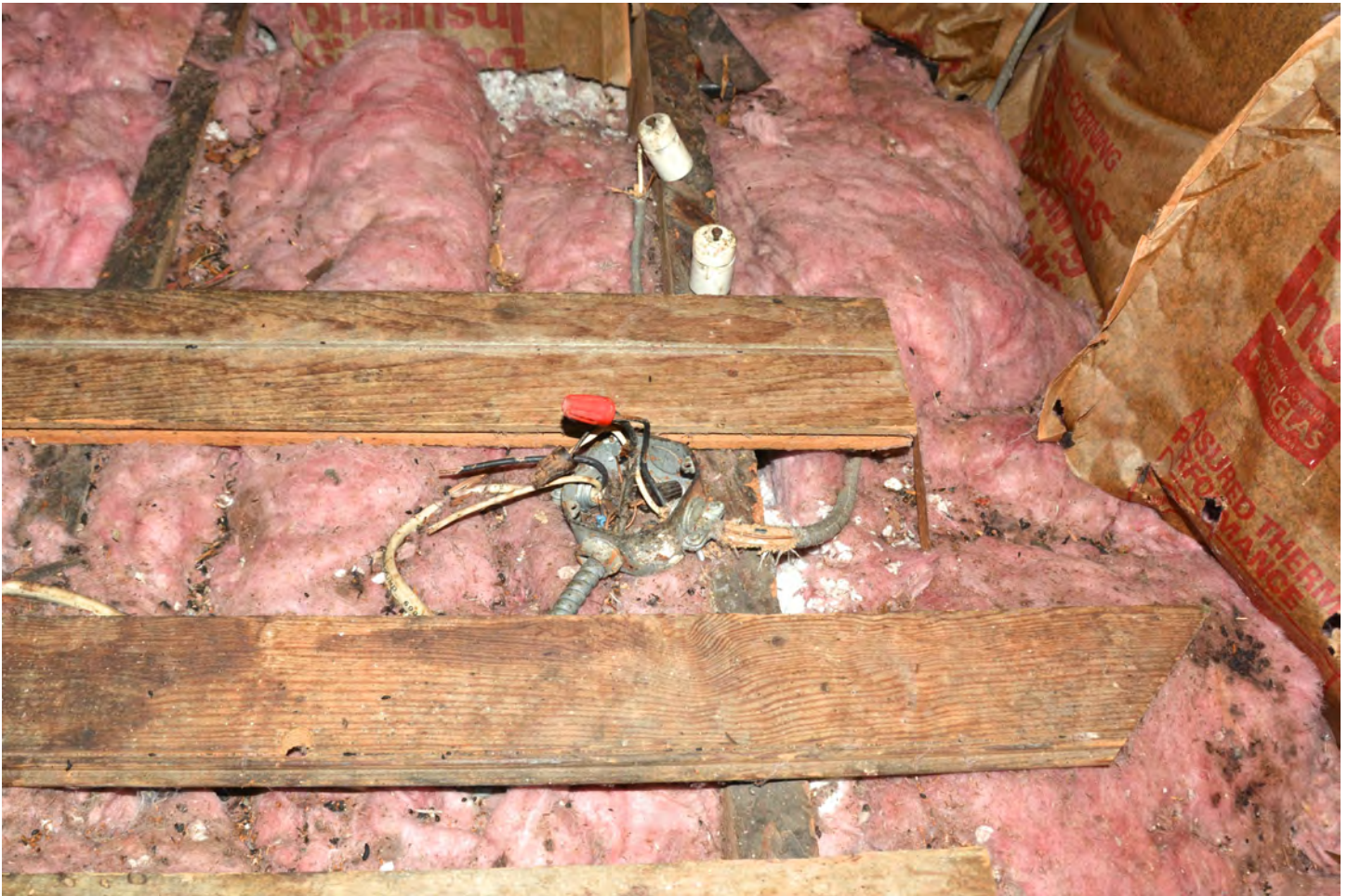
This is a junction box located above the closet ceiling that is also missing a cover. Notice how the wiring insulation has been chewed away exposing the copper wire. There is also a black grounding wire that is not connected to anything.
