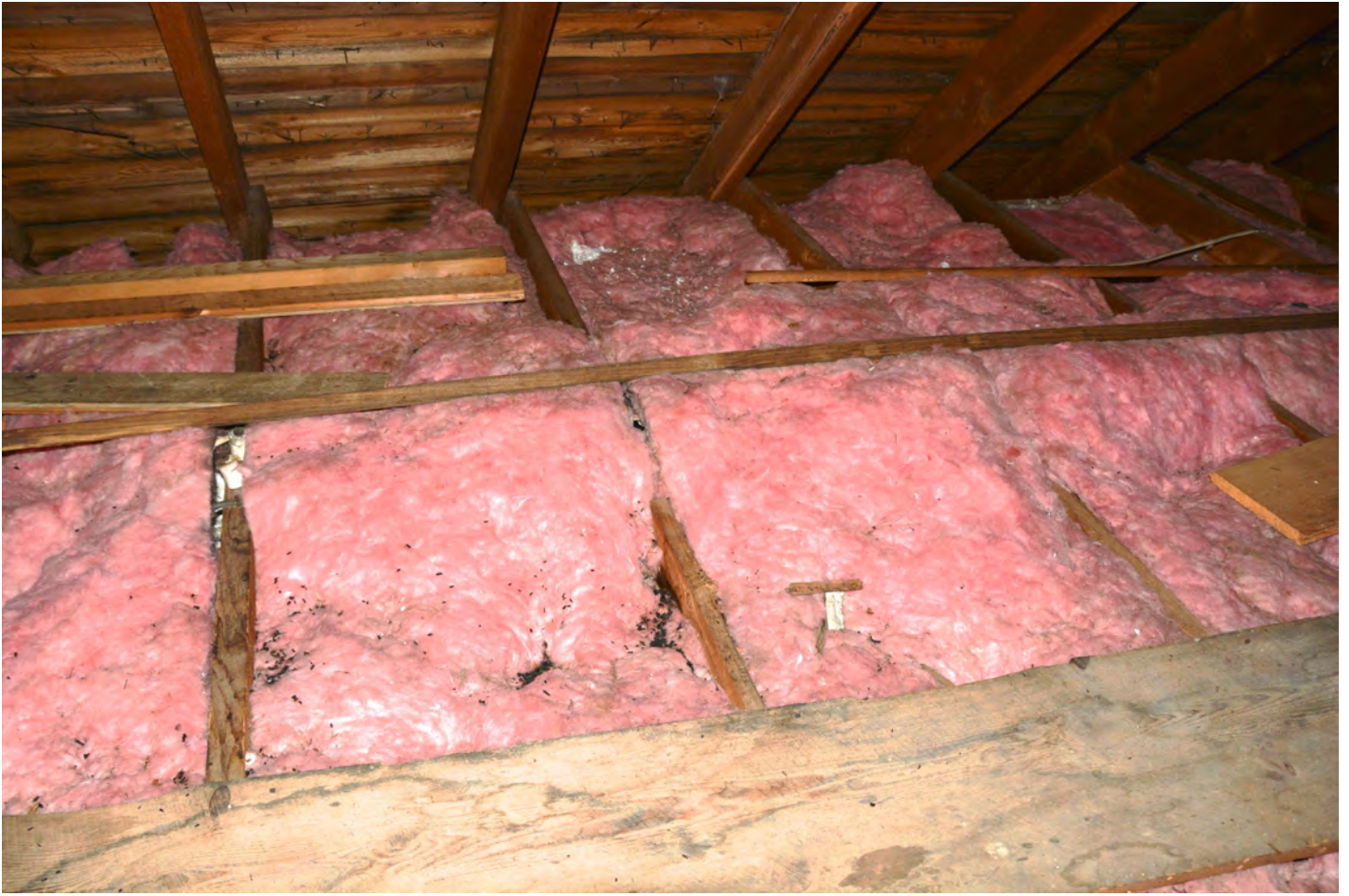
Attic area to the north of the building. Again, notice the animal waste on top of the insulation and the 'hump' where the insulation was placed on top of electrical wires.
