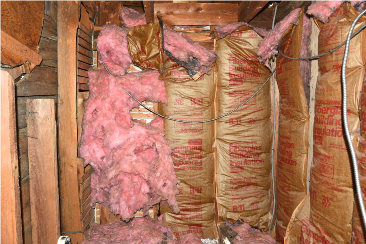
This is the attic area above the closet. As you can see, wall insulation is falling down and needs to be replaced.
