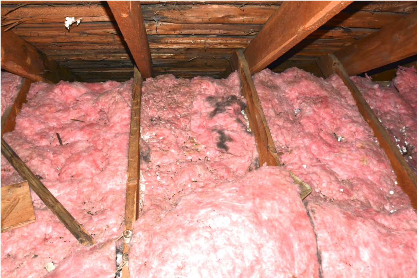
This is the area above where the stain was identified in the ceiling. Note the animal fur in the center of the picture and how the insulation in this section is matted down. Also note the electrical wires that are nailed to the top of the ceiling joists in the bottom left corner of the picture and how the insulation was placed directly on top of it.
