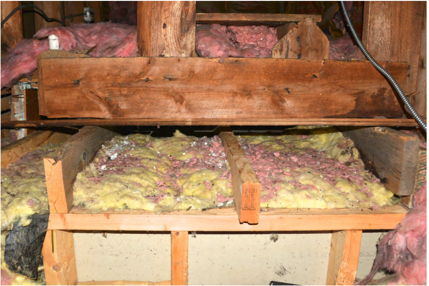
This is the ceiling above the entryway to the museum. Notice how the mice have chewed away pink insulation and scattered it over the yellow insulation. Also notice how the yellow insulation has been matted down as a result.
