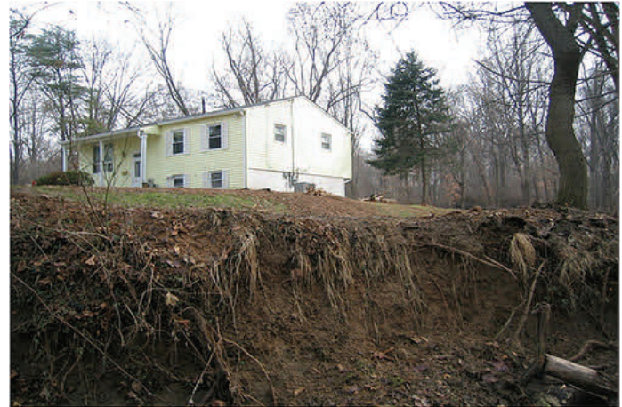
Examples of the damage storm water runoff can cause.
