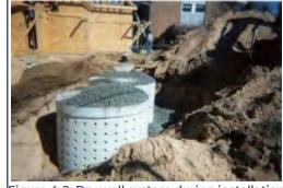
Figure 4-2: Dry well system during installation
