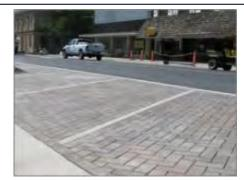
Figure 4-1: Permeable paving system
