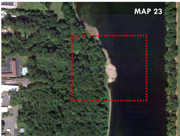
Photo: Tannery Brook Erosion in the Connecticut River/Google
