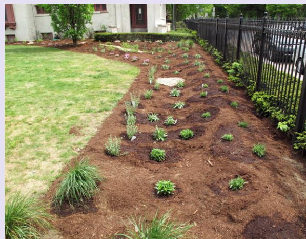
Rain gardens gather and sink water instead of entering stormwater drains that pollute the Ct. River watershed. Photo courtesy of Regenerative Design Group.
