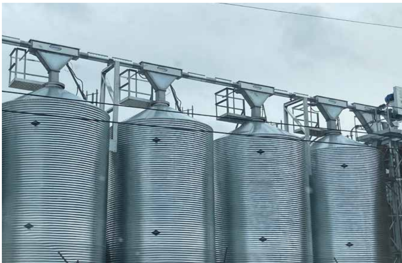
Valley Malt Grain Silos
