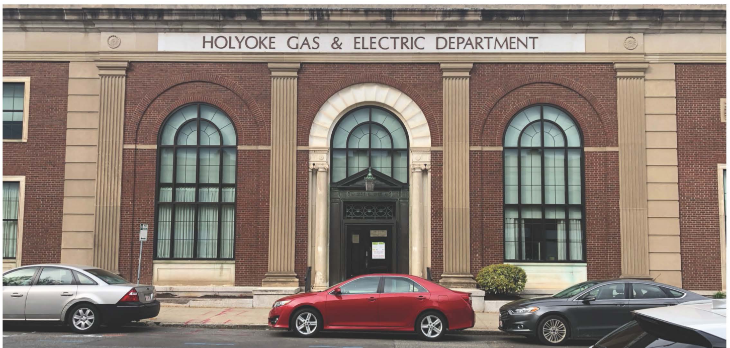
Image of Holyoke Gas and Electric Department. Photo Credit: Third Eye Network
