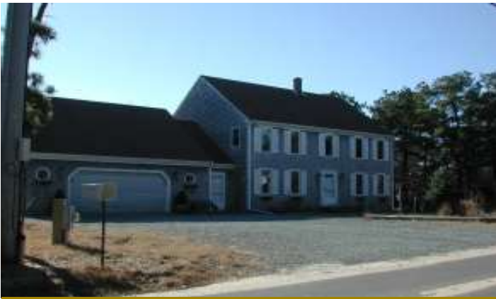
Interior ADU – Town of Wellfleet Photo credit: Town of Wellfleet
