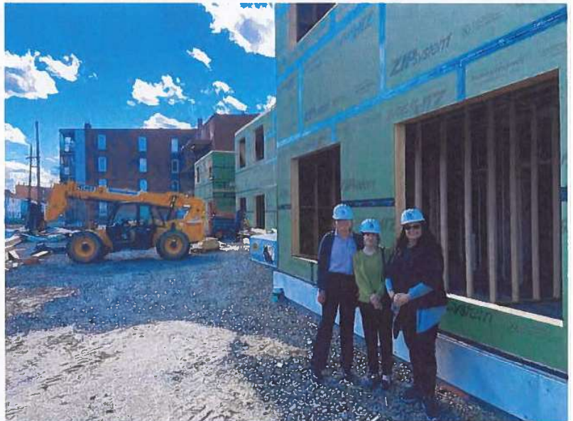
HRA Board and staff tour the Phase 1 site
