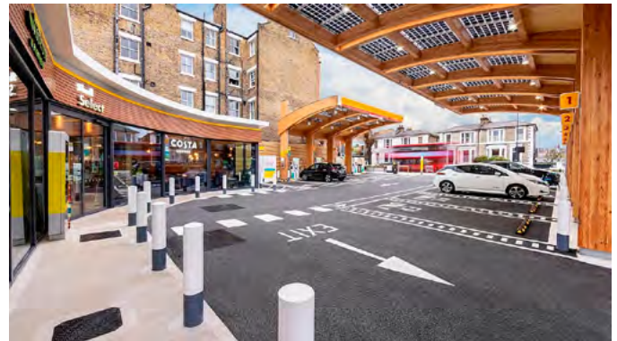
Figure 73 - Shell Solar Station in London, UK. (Source)
