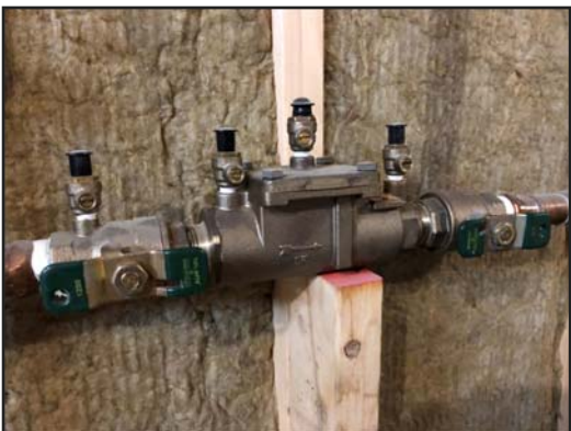
Residential Backflow Device Protects Drinking Water Supply
