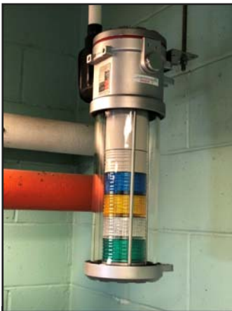
New Multi-Color Alarm Strobes
