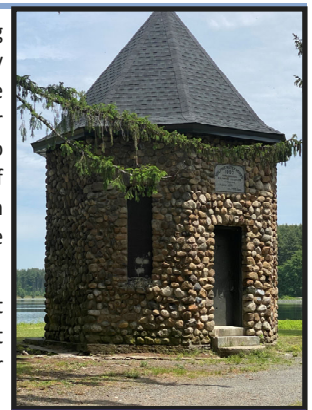
Ashley Reservoir Gate House
