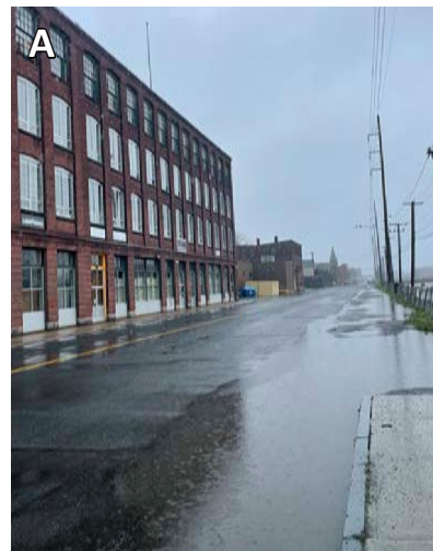
Pooling on the edge of Race Street along the canal.
