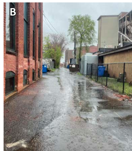
Pooling along the back alleyway between Main and Race Streets.
