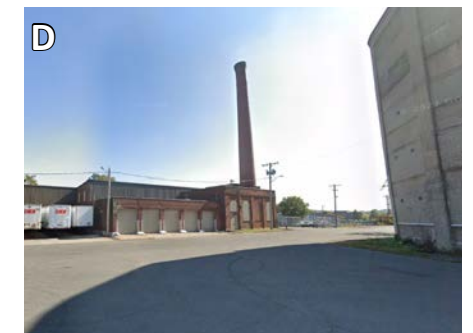
Crescent and Clement large paved intersection.
