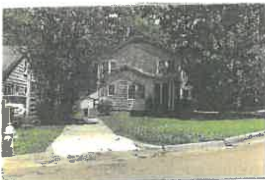
West Side View of Duplex
