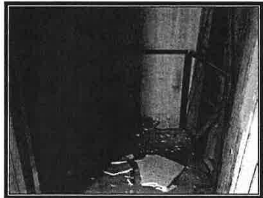
DUMB WAITER ELEVATOR SHAFT
