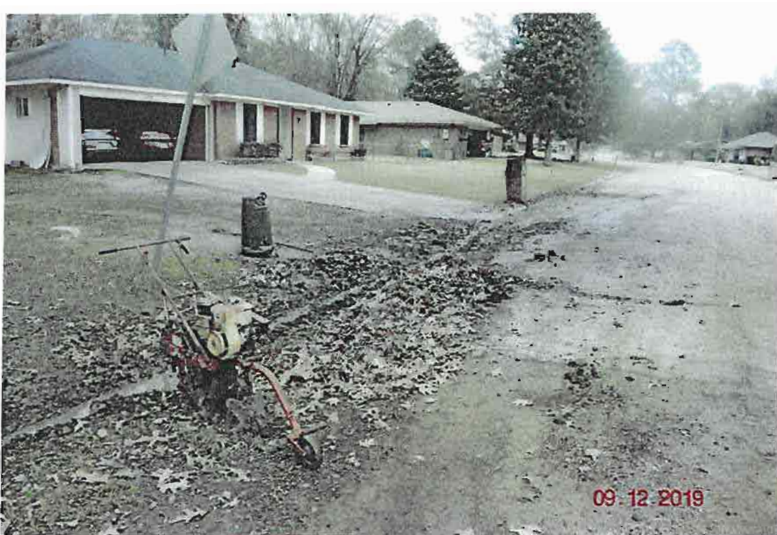
Drainage ditches downhill blocked causing neighbors to clean out concrete gutters.
