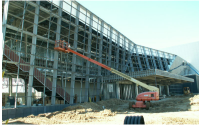
JACKSON CONVENTION CENTER CONSTRUCTION
