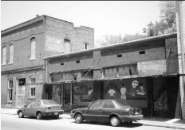
New construction should present a one- or two-story facade at the front property line.
