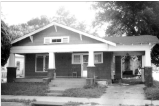
A porte cochère may be considered as an alternative to a garage.
