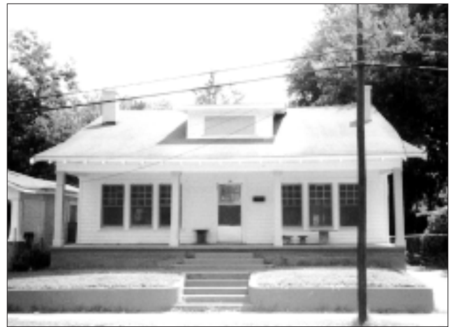
In many areas, houses were elevated above the level of the street due to the hilly terrain. Where this occurs retaining walls were typically used.
