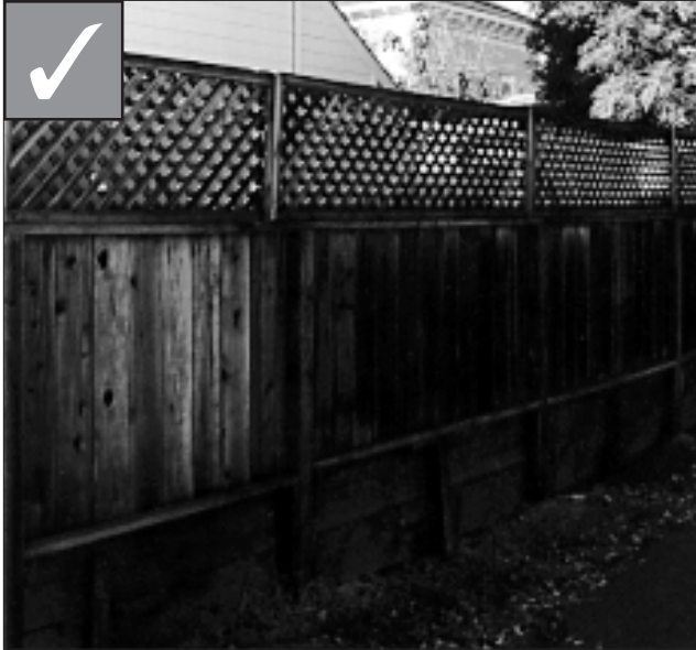
Consider using lattice, or other transparent detailing, on the upper portions of a side or rear yard fence.
