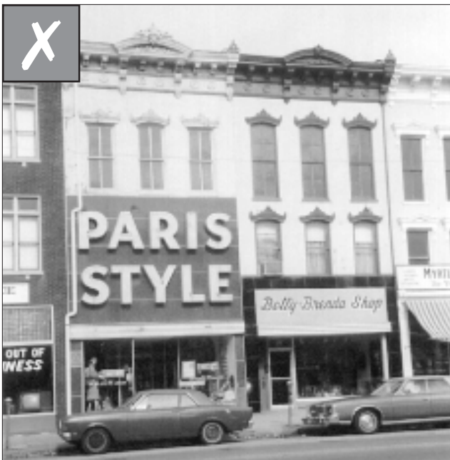
Any sign that visually overpowers the building or obscures significant architectural features is inappropriate.
