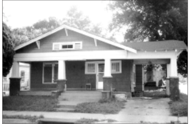
An attached carport, known as a porte cochère , provided a covered parking area adjacent to a house.
