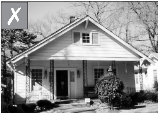
This porch has undergone an alteration that is not appropriate; wrought iron supports have replaced wood piers.
