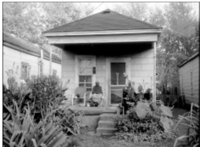
Although there is not much applied architectural detail seen on this Shotgun, its narrow and long rectangular form is a distinguishing feature that should be preserved.
