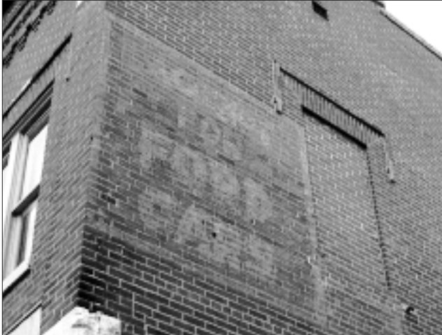
Existing painted “ghost” signs should be maintained when feasible. A ghost sign should not be coated with varnish or polyurethane, but rather touched up as needed.
