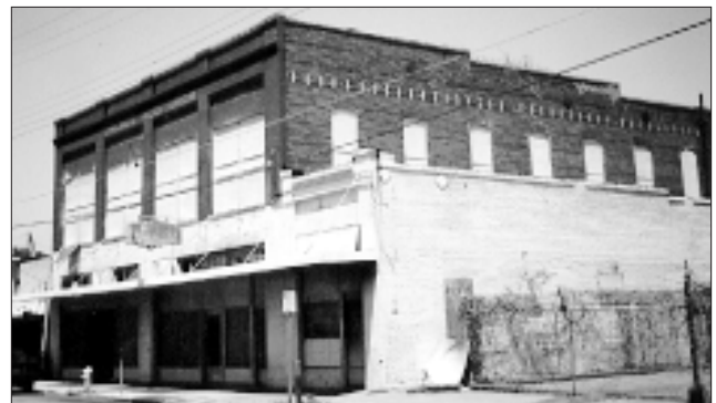
The arched windows, corbelled brick and cornice moldings contribute to the character of the street.
