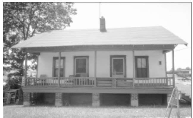
The Creole Cottage features a full-length porch with simple detailing.
