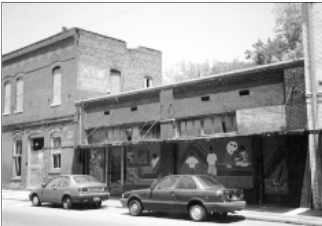
The commercial buildings relate to a human scale since they don't rise above two stories.
