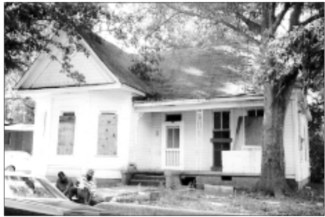
L-Front Cottage houses feature a front facing gable portion and a side-gabled wing that connect to form an L-shaped plan.
