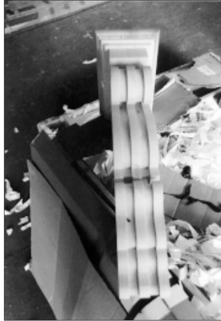
Replace features that are missing or beyond repair. Reconstruct only those portions that are damaged beyond repair.
