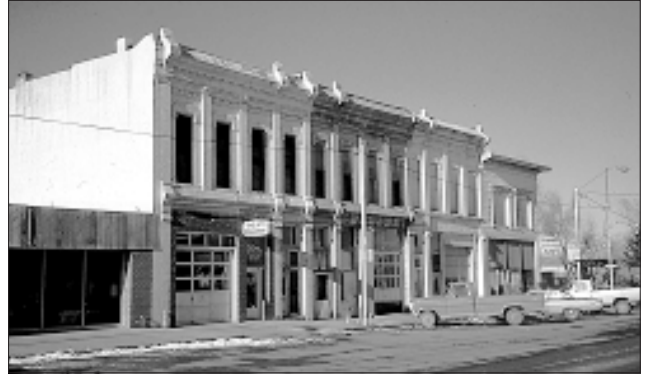
In this photo, the row of buildings has lost architectural detail over time and a monochromatic color scheme obscures the original design character.
