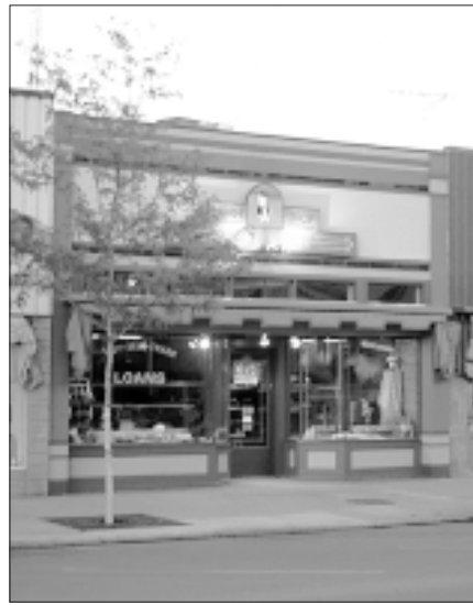
The same building (at left) after renovation, exhibits the more classical features, including a painted cornice, kickplate and recessed entry.
