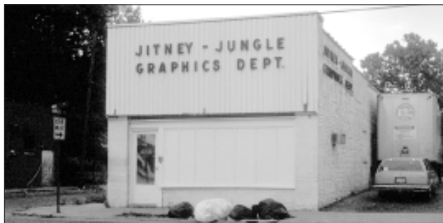
All of the buildings in the commercial core are brick. This building has been partially covered with another material.
