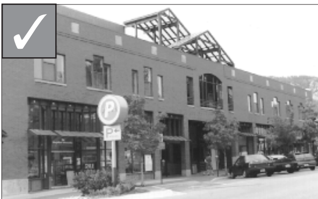
Design a parking structure to allow space for active uses at the sidewalk edge.
