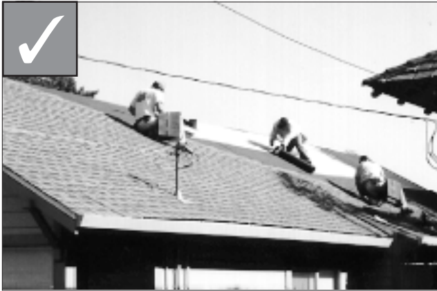
Composition shingles are an acceptable roofing material.
