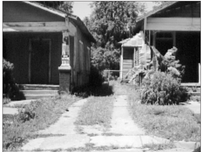
Also consider using concrete strips that lead to the garage. This would further reduce the driveways visual impacts.
