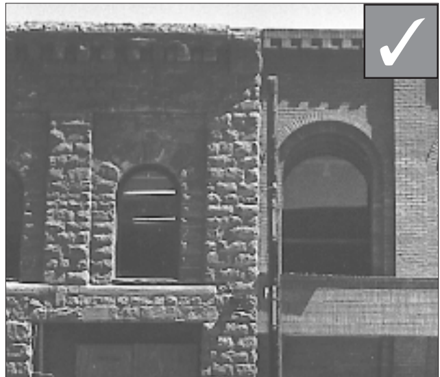
Materials should be similar to those used traditionally. Although not built with stone, the newer building (right) uses a similarly colored masonry material to the historic building (left).
