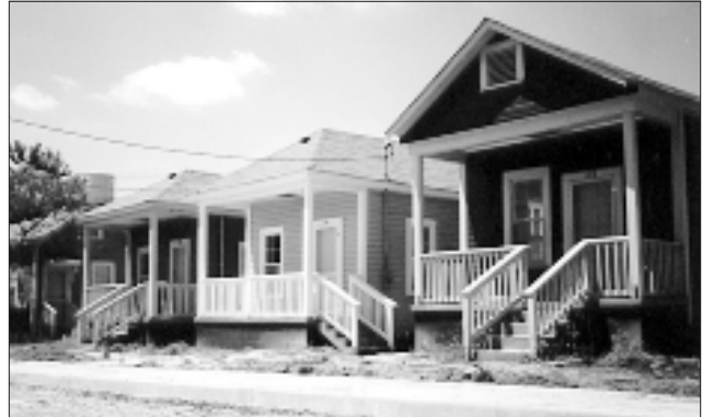
Shotgun houses are typically one room wide and two or more rooms deep, with no hallway.
