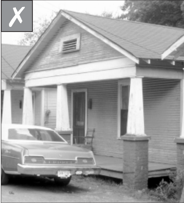
Parking in the front yard of a residence is inappropriate.
