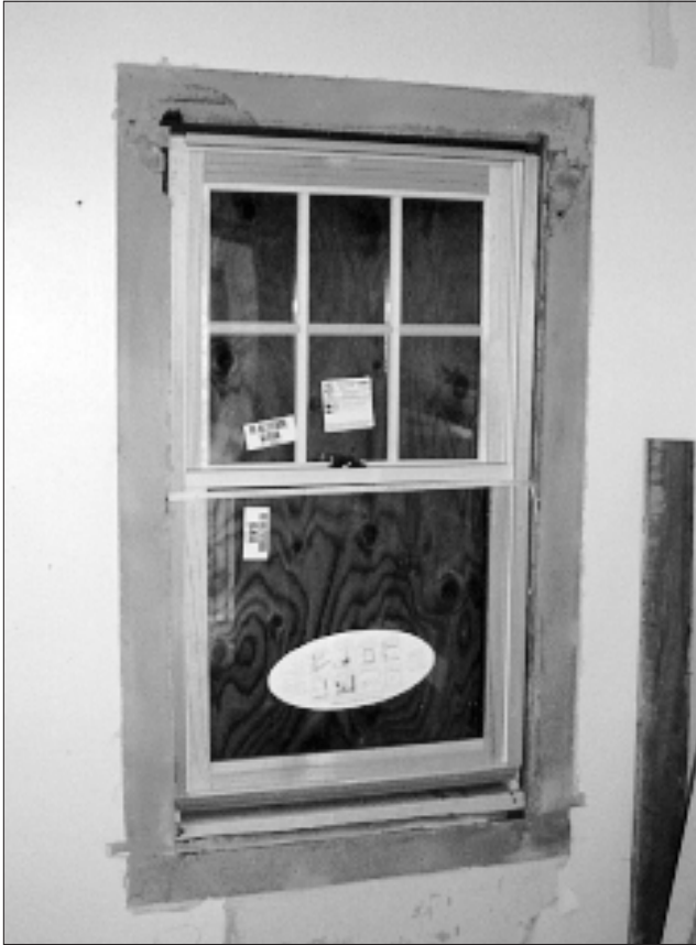
In a replacement window, use materials that appear similar to the original. Wood is the preferred material.
