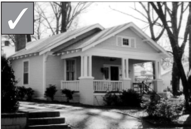
When considering a new porch, design it to be similar to those seen historically. This porch construction was based on neighboring houses of similar character and age.
