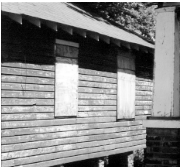
Good preparation is key to successful repainting, but the buildup of old paint layers is an important historic record of the building. The removal of old paint, by the gentlest means possible, should be undertaken only if necessary to the success of the repainting.
