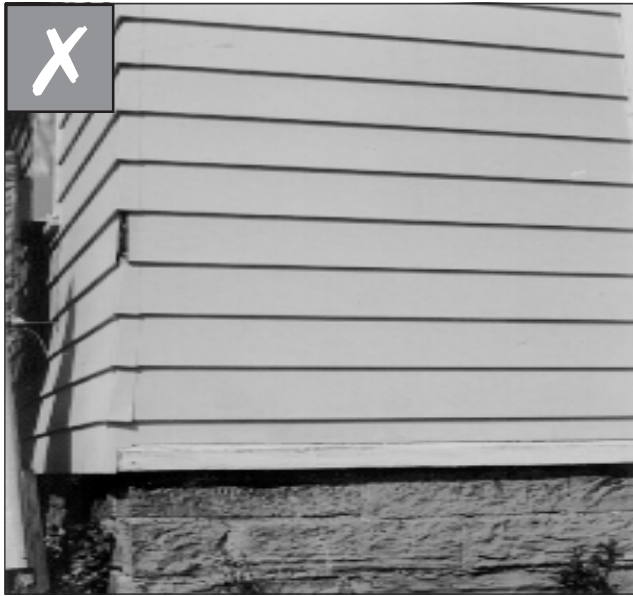
Consider removing inappropriate covering materials; examples include vinyl, aluminum or asphalt siding.
