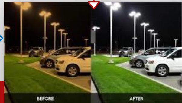
LED Lighting – Before & After
