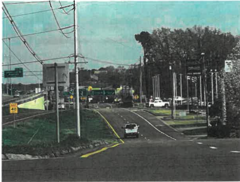
Photograph from Frontage Road (facing northbound) depicting tall trees blocking the property from view on righthand side
