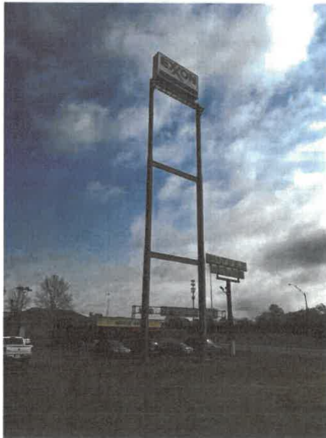
Photograph of high-rise Exxon sign at Northside Drive exit—just two exits from the planned QuikTrip
