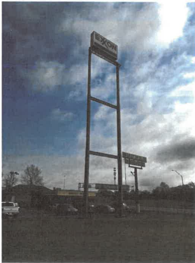
Photograph of high-rise Exxon sign at Northside Drive exit—just two exits from the planned QuikTrip
