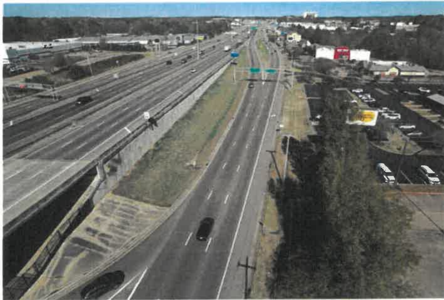
Drone photograph showing Cracker Barrel sign not visible from I-55 S due to trees
