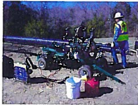
Polyethelene Pipe Joints being Fused Together
