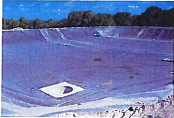
Backwash Holding Pond
