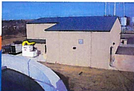
South End of 3 MGD Water Treatment Plant Building, Emergency Generator, Chlorine Scrubber
