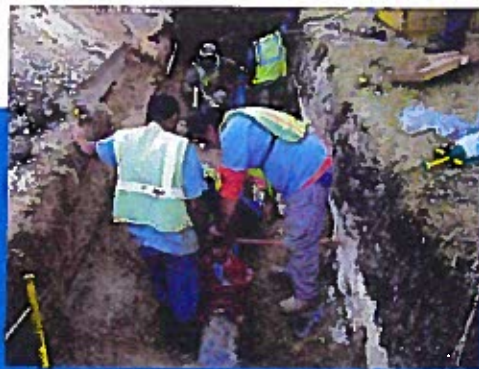
Gate Valve being Set in Place on Polyethelene Pipe
