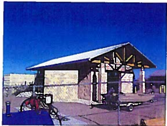
Electrical and Control Building at Lake Stillhouse Hollow Raw Water Intake Site
