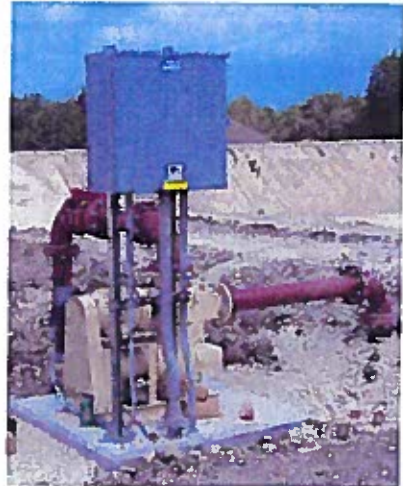
Supernatant Return Pump Station
