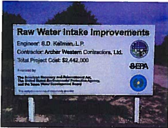
American Recovery and Reinvestment Act Sign at Raw Water Intake Site
