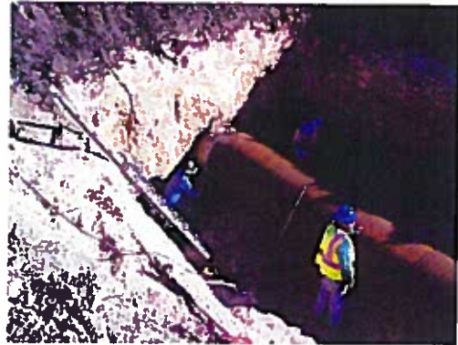
Water Line Bore under Highway
