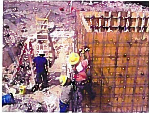
Form and Rebar Work on Walls of Surge Relief Valve Vault
