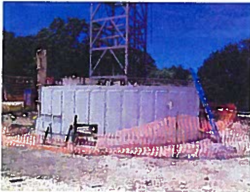
Lower Concrete Support Wall Structure
