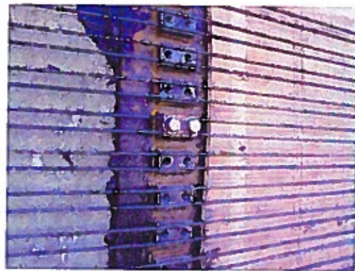
Reinforcing Steel on Walls of Clearwell during Construction of Tank
