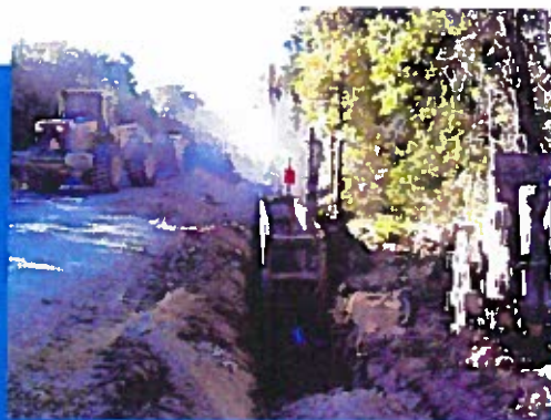
30" Water Line under Construction
