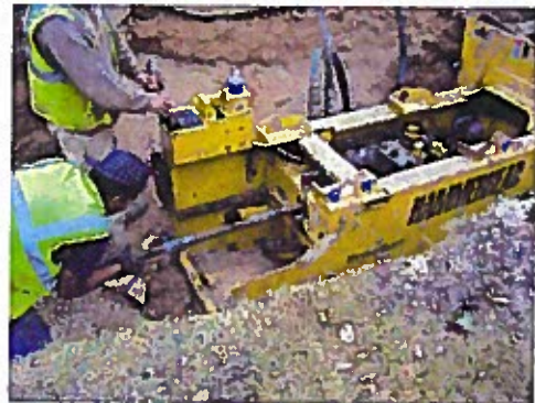
Pipe Burst Machine in Trench
