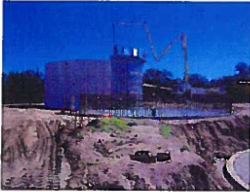
Two Concrete Clarifiers under Construction
