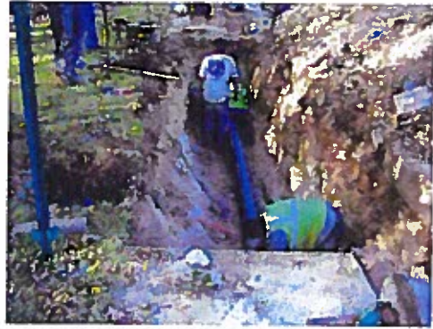
Polyethelene Pipe in Trench
