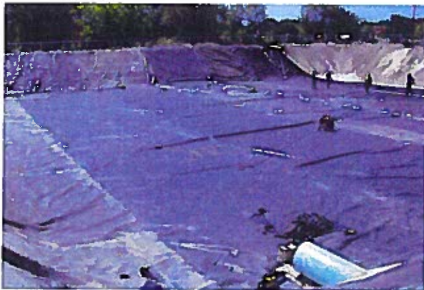
Backwash Holding Pond
