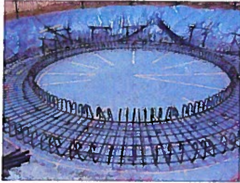
Foundation under Construction
