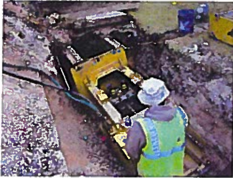
Pipe Burst Machine in Trench
