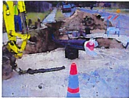
Plug in Polyethelene Pipe; Pipe Burst Procedure Saves Existing Sidewalk
