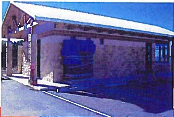
Electrical and Control Building at Lake Stillhouse Hollow Raw Water Intake Site
