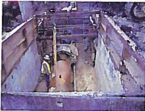
Water Line Bore under Highway
