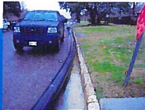
Polyethelene Pipe Sitting on Pavement
