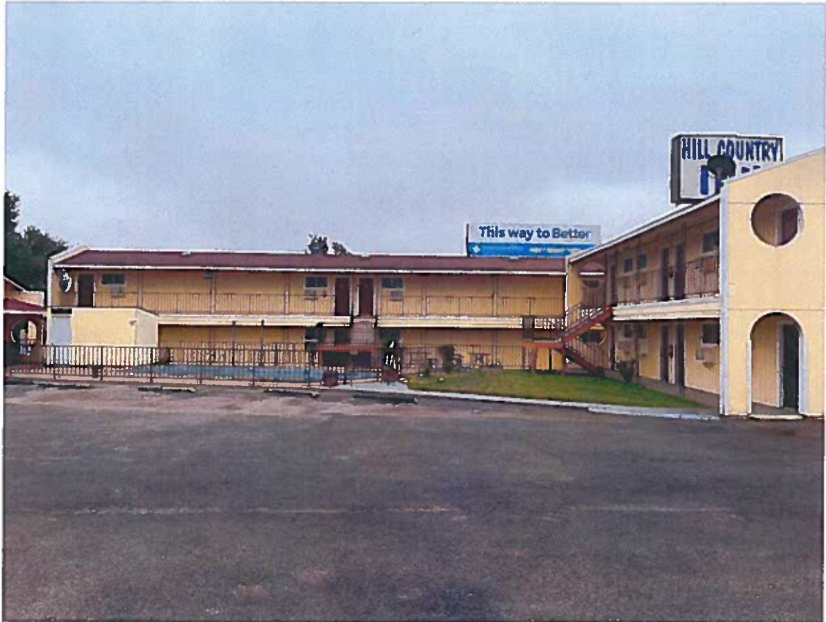
Building B & C:
