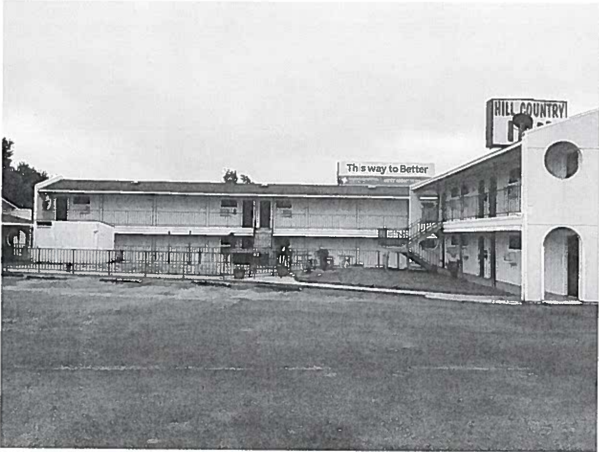
Building B & C:
