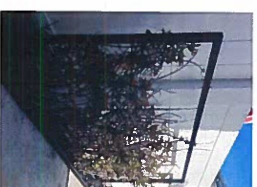
Plant Trellis on left exterior of building
