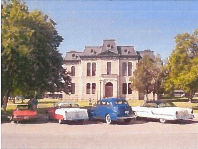
Figure 3-2: Old Blanco County Courthouse, City of Blanco
