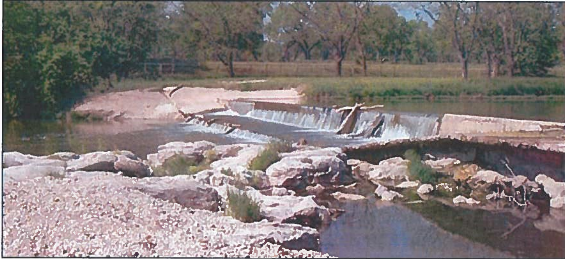
Figure 16-1 Lake Johnson City Dam
