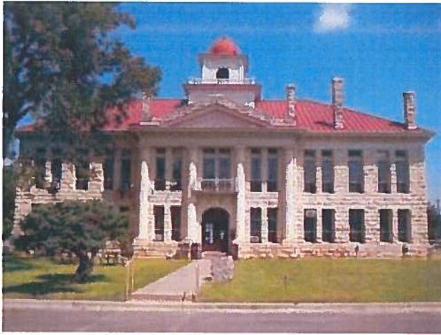
Figure 3-2: Blanco County Courthouse, Johnson City
