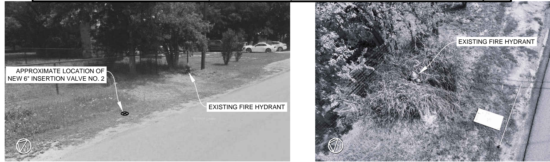
FIRE HYDRANT NO. 8 REPLACEMENT, INSERTION VALVE NO. 2 INSTALLATION (Old Austin Highway at Mesquite)
